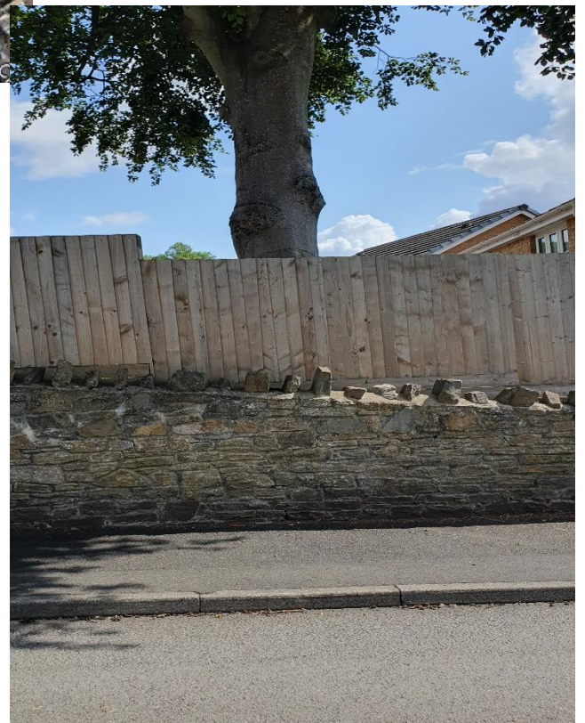
Photograph 2. Boundary wall and Fence
