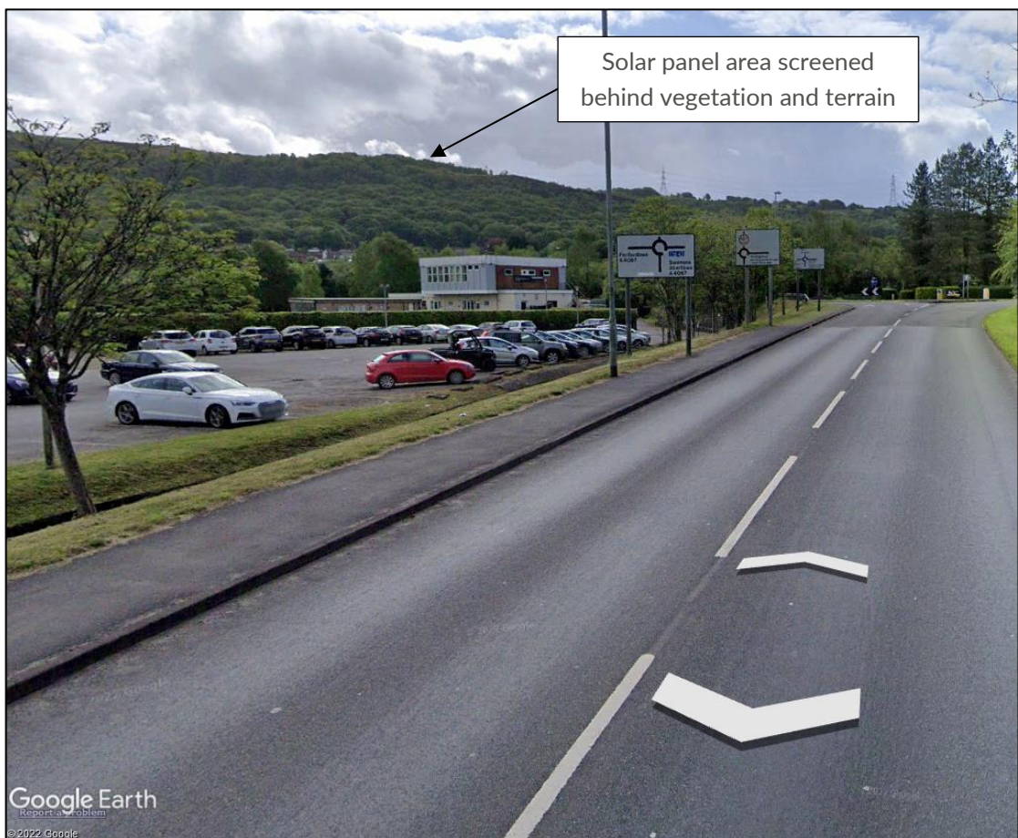
Figure 31 Street view image from receptor 15, showing the views towards the reflecting panel area
