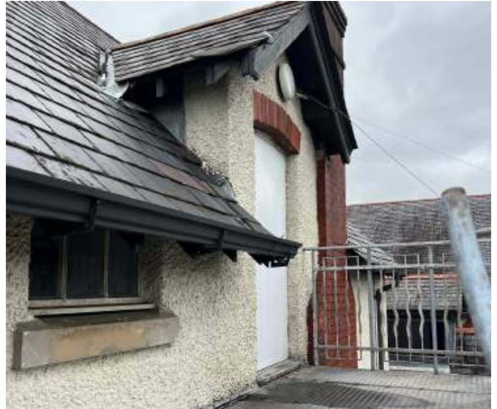
Photograph 138: Slate roofed dormer providing external fire escape onto spiral stair. The stair is modern however it is not clear whether the current stair replaced an earlier stair or whether the dormer was previously a window that has been reconfigured to a door. The brick arch appears contemporaneous with others on the building suggesting that may be original.
