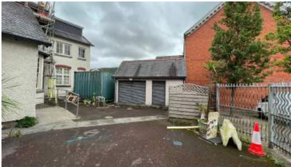
Photograph 136: View towards back of theatre with sash windows and modern plant room dormers
