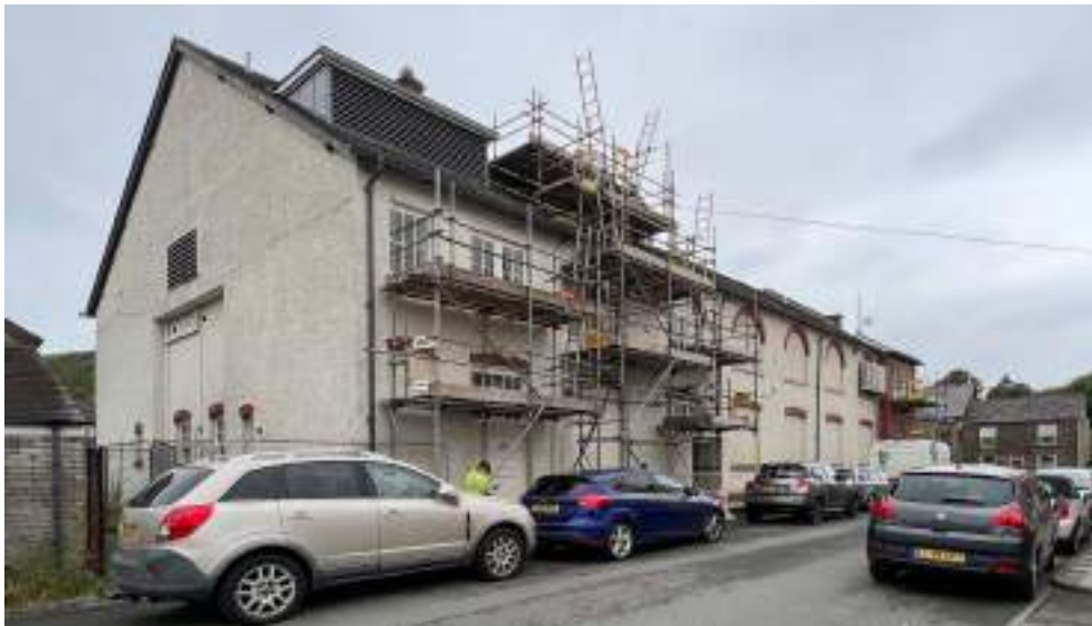
Photograph 131: Sash windows to the rear dressing rooms and other supporting spaces with modern flat roofed dormers housing the plant room above
