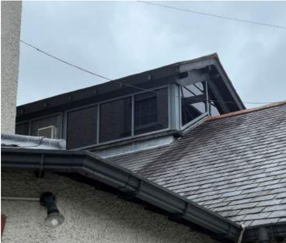
Photograph 139: Original glazed roof lantern situated over the bar area. Lantern has a pitched slate roof with glazed sides. The glazing appears to be modern so is likely a replacement of the older timber windows
