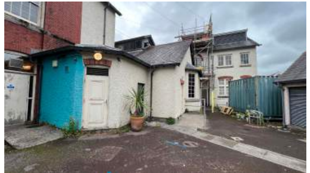
Photograph 137: Service space with arched brick door head between cafe to the left and studio space to the right
