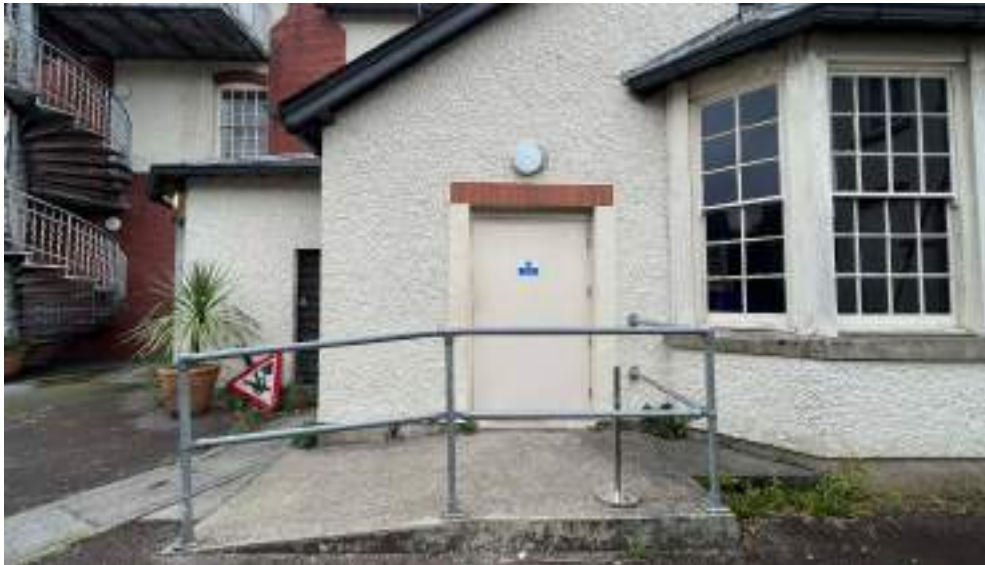
Photograph 134: Brick head to door appears to be modern, assumed to have been added in 1996 to provide a new fire escape to studio
