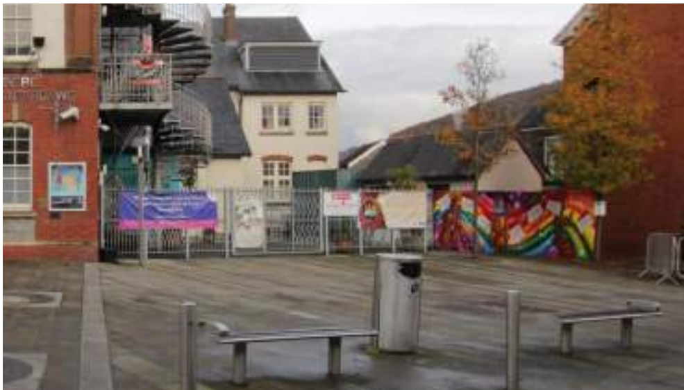
Photograph 119: To the right hand side of the building is a courtyard which is enclosed with a modern brick wall with mural artwork and galvanised steel palisade fence and gates. The age of these are unknown but unlikely to be older than the 1996 conversion.
