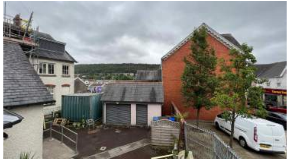
Photograph 135: View from top of spiral stair of neighbouring gable ended building and flat roof dormer to rear of auditorium for plant room
