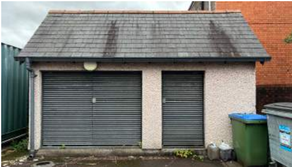
Photograph 129: Modern rendered blockwork plant room with slate roof
