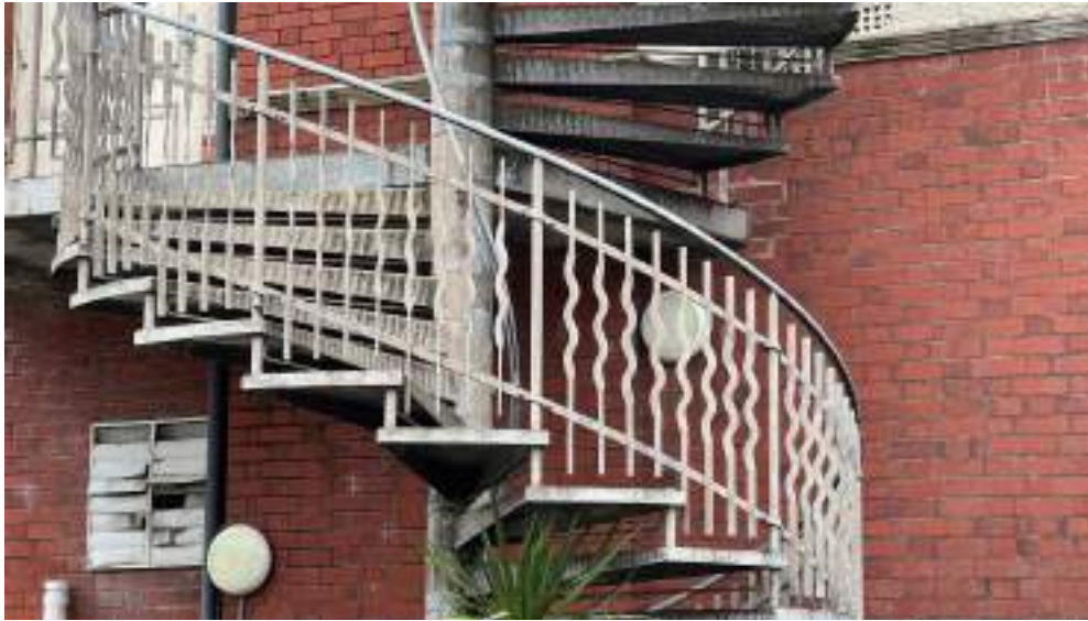
Photograph 128: Modern galvanised steel spiral escape stair in front of brick walls
