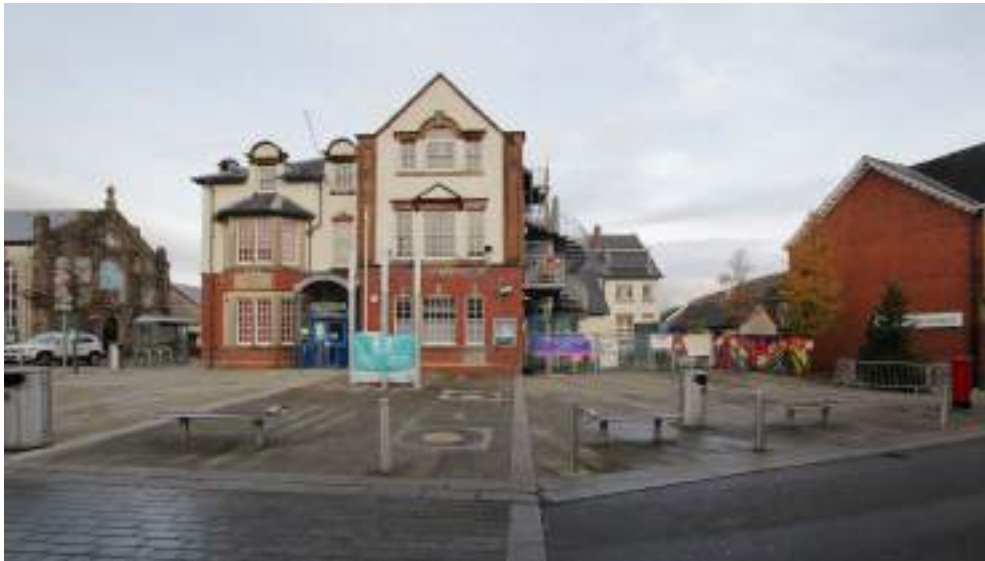
Photograph 117: Principal elevation as viewed from Herbert Street
