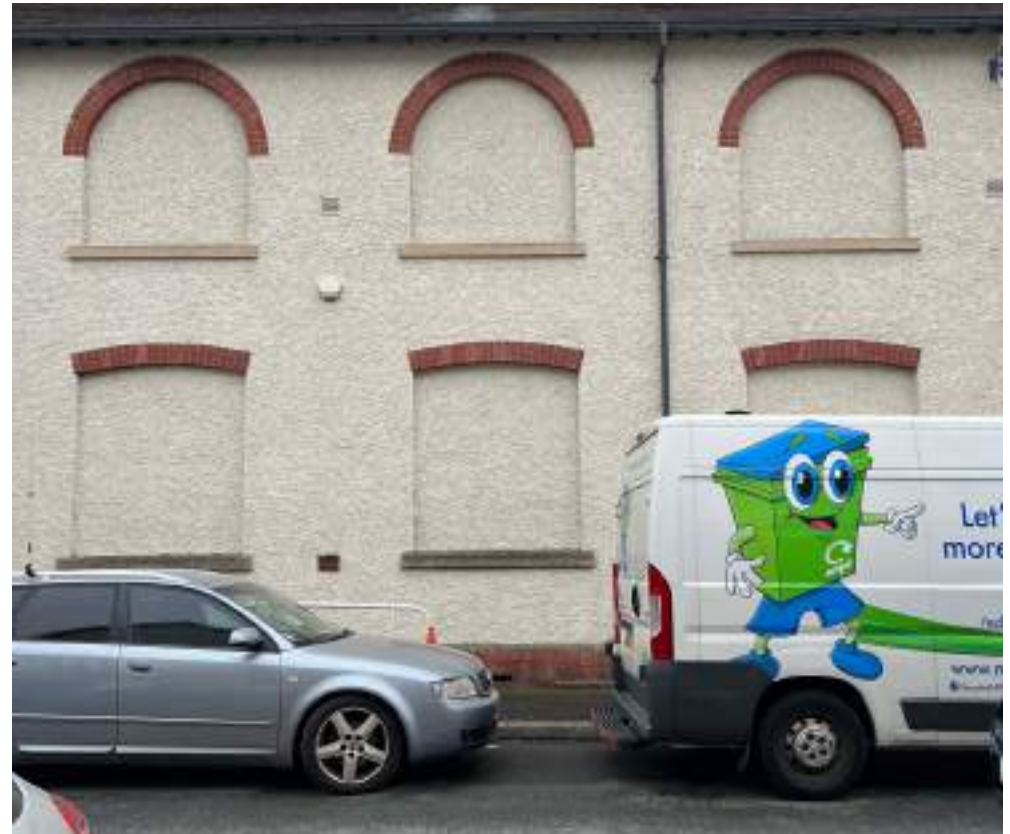
Photograph 128: Series of brick arched recesses along the auditorium portion of the south eastern facade
