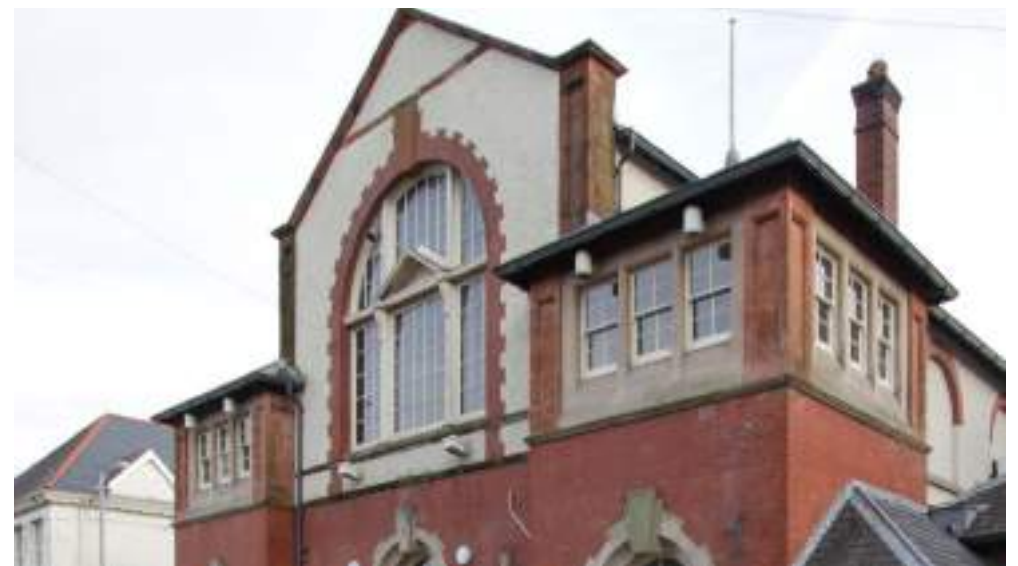
Photograph 127: The eastern most volume housing the auditorium with its central gable with brick arch surround and flanking volumes housing the staircases
