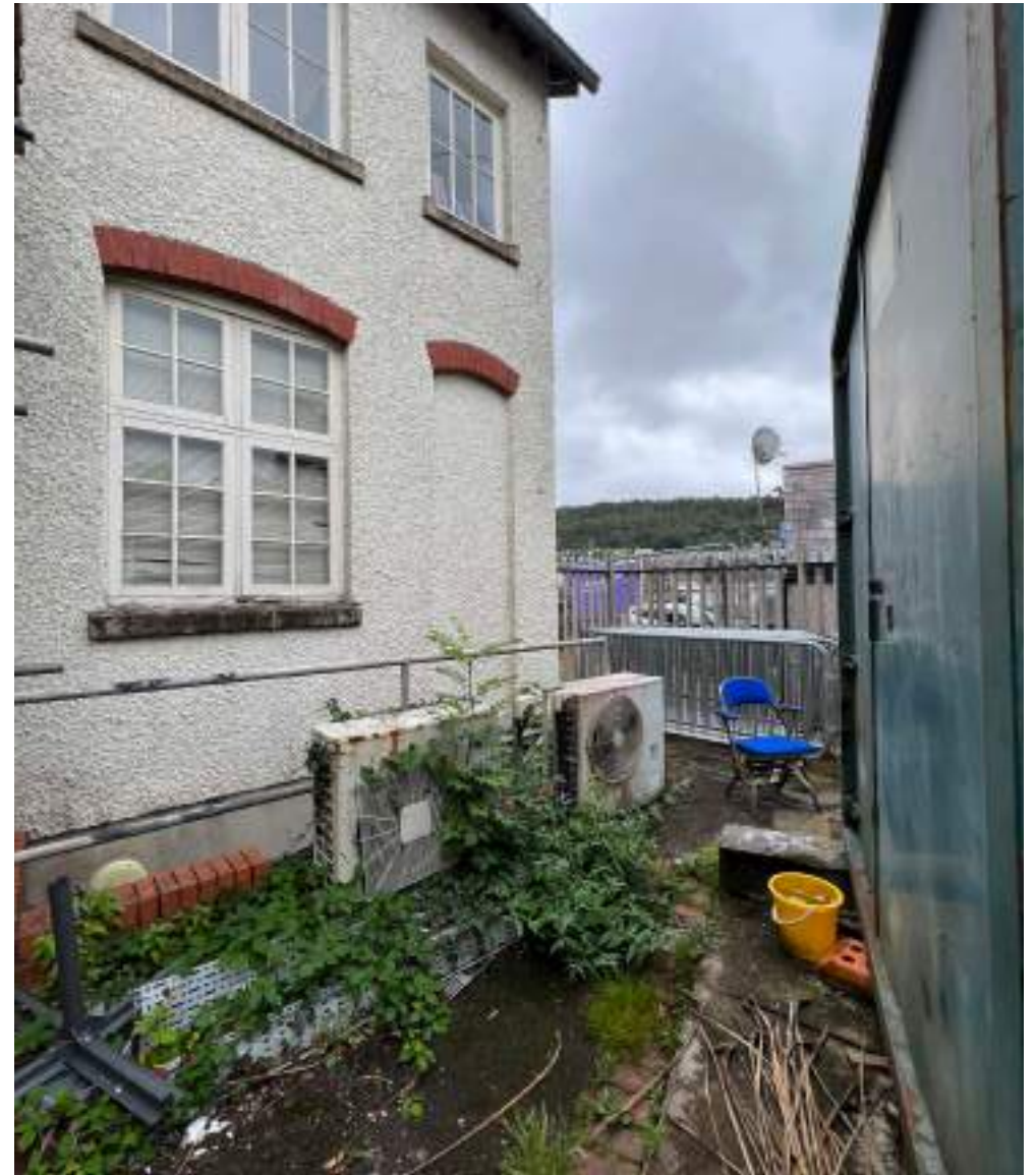
Photograph 125: Timber sash windows with brick arched heads and mechanical plant and shipping container to the right
