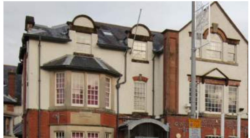
Photograph 120: Mix of bay windows and flat window triptychs with arched rooflights
