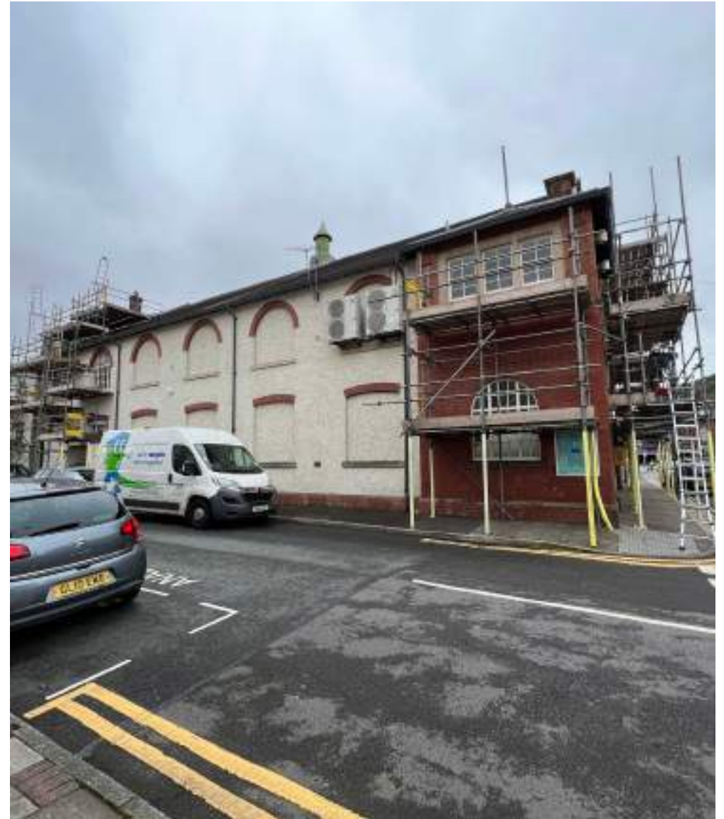
Photograph 130: Brick corner sections housing the main internal staircases leading up to the first floor of the auditorium
