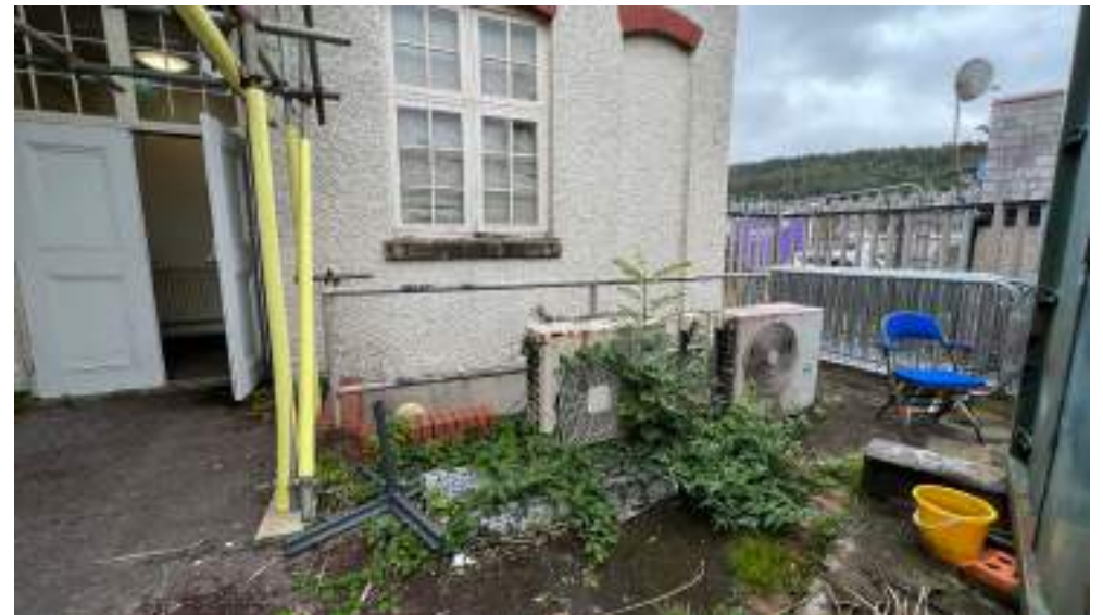
Photograph 123: Fire escape from theatre and timber sash windows
