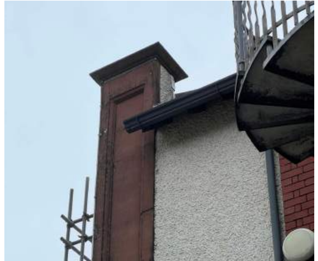
Photograph 140: Carved stone parapet wall detail with decorative stone coping
