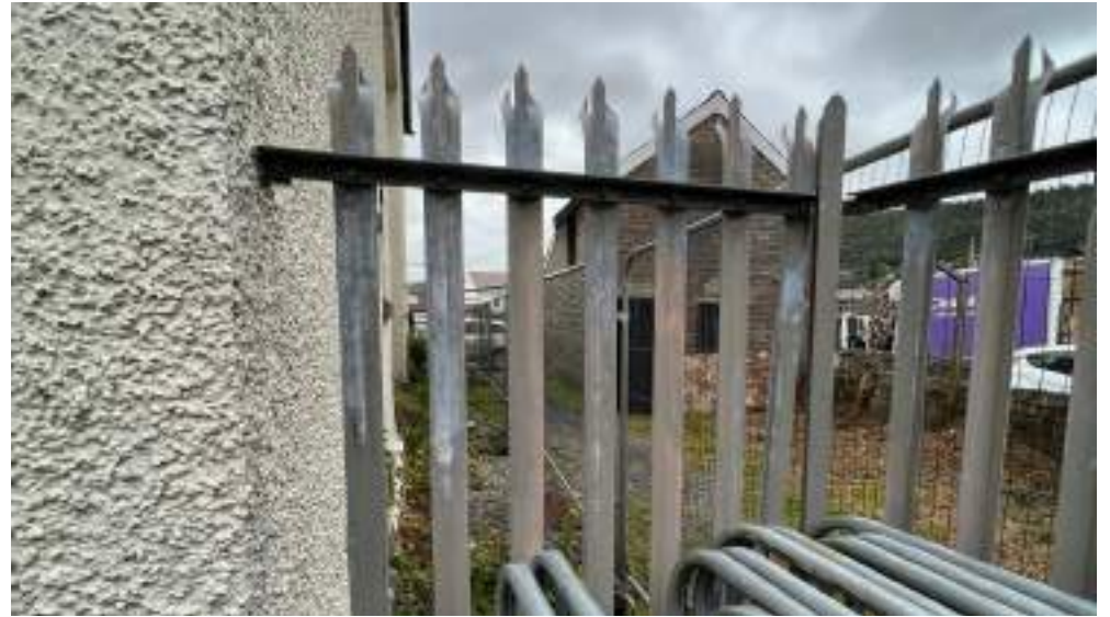
Photograph 126: Modern galvanised palisade fence to perimeter of courtyard
