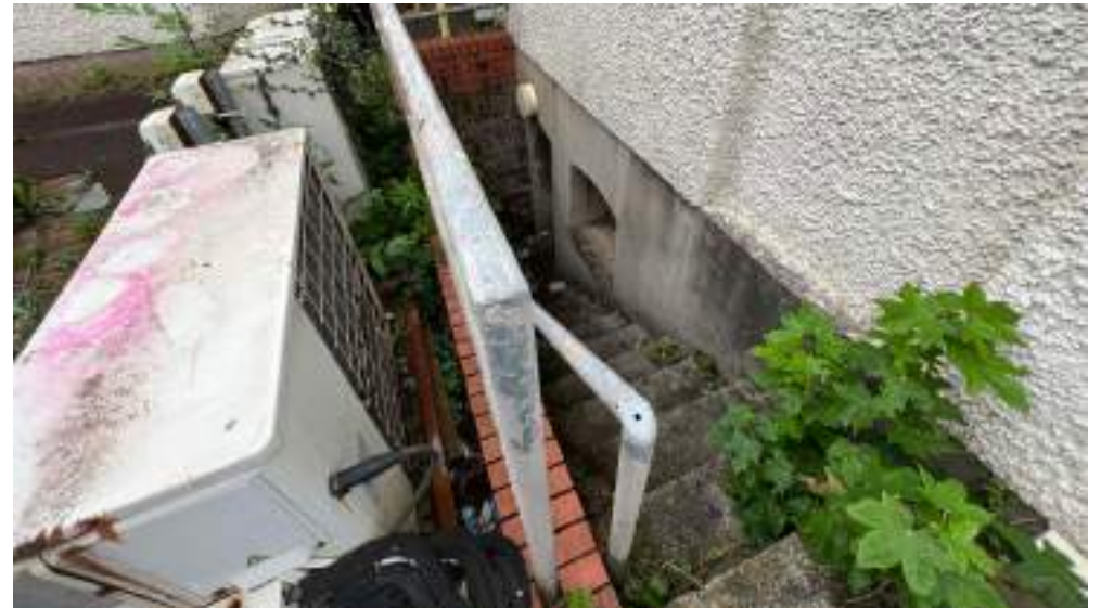
Photograph 141: Steps leading down to basement below theatre
