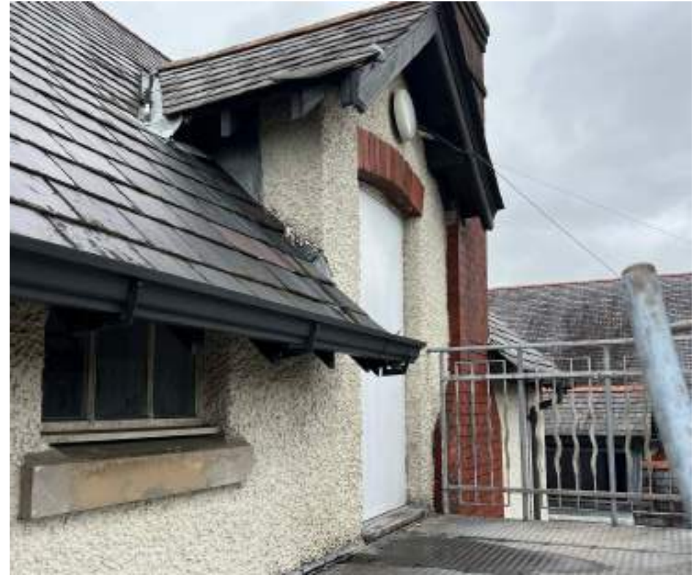
Photograph 130: Slate roofed dormer providing external fire escape onto spiral stair. The stair is modern however it is not clear whether the current stair replaced an earlier stair or whether the dormer was previously a window that has been reconfigured to a door. The brick arch appears contemporaneous with others on the building suggesting that may be original.
