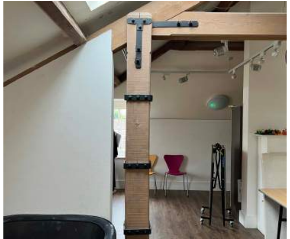
Photograph 106: A-framed timber roof trusses with black metal bolted straps
