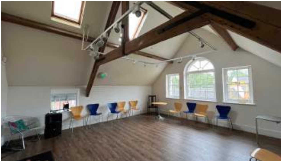
Photograph 109: Original timber sash windows and central arched window
