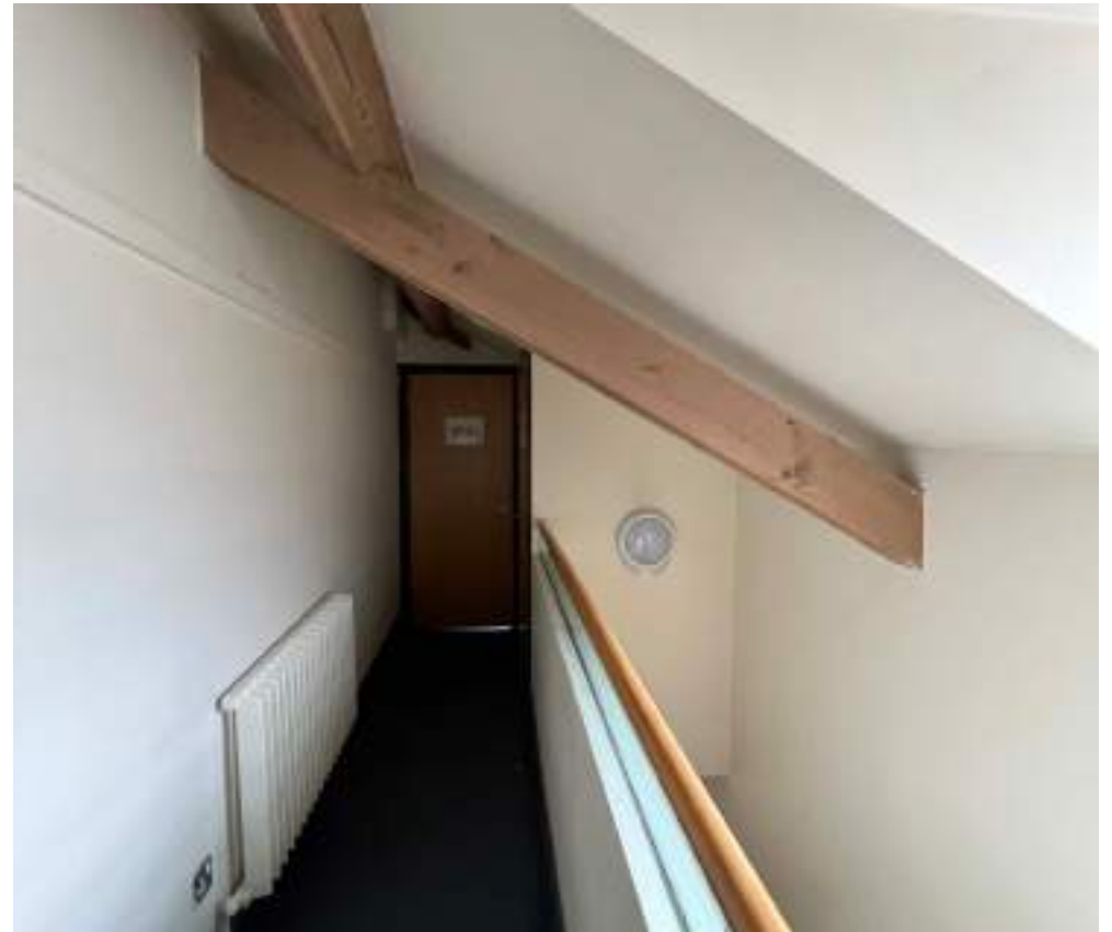
Photograph 101: Modern stair case with original timber roof structure exposed
