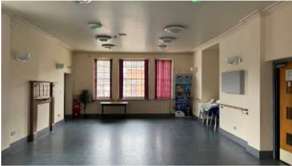
Photograph 93: Timber sash windows, fireplaces and cornice with modern doors
