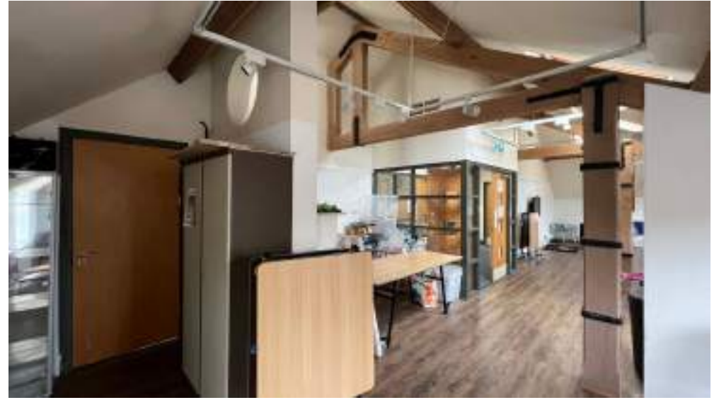
Photograph 108: A-framed timber roof trusses and modern stud partitions
