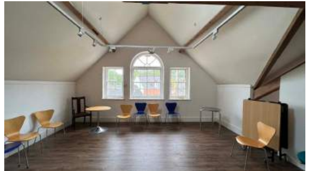
Photograph 110: Original timber sash windows and central arched window
