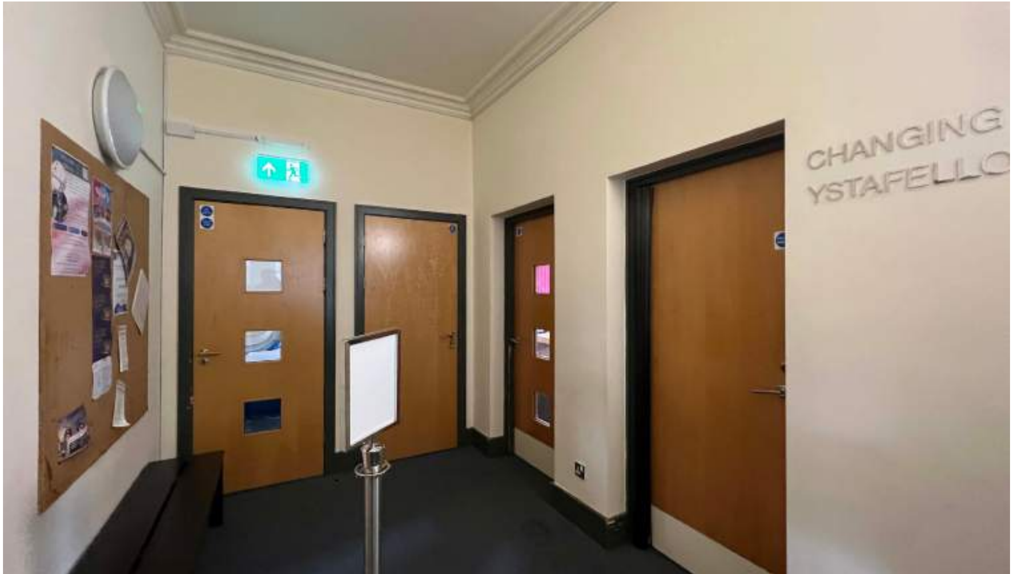
Photograph 87: Modern finishes and doors with historic cornice
