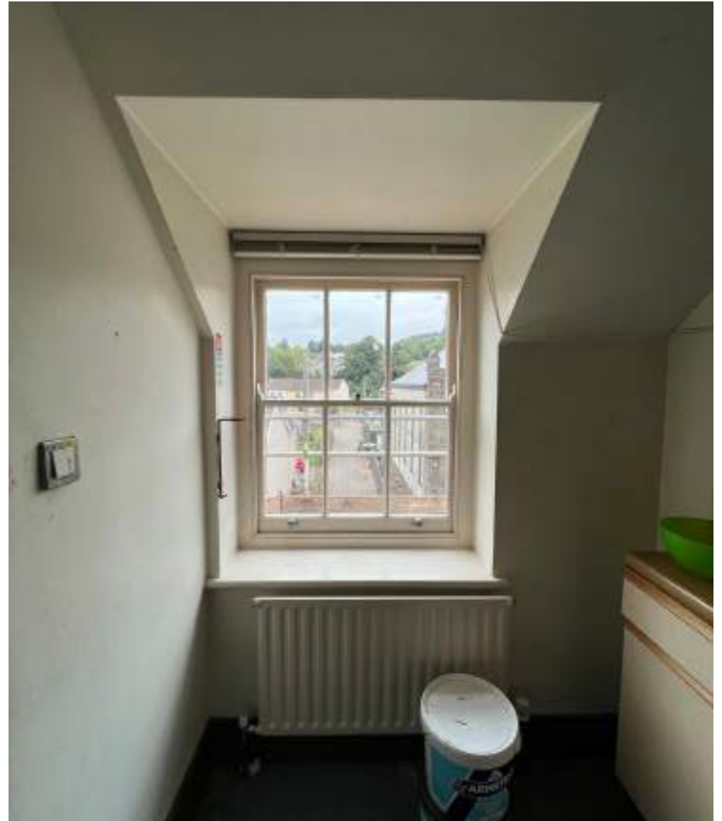
Photograph 113: Timber sash window
