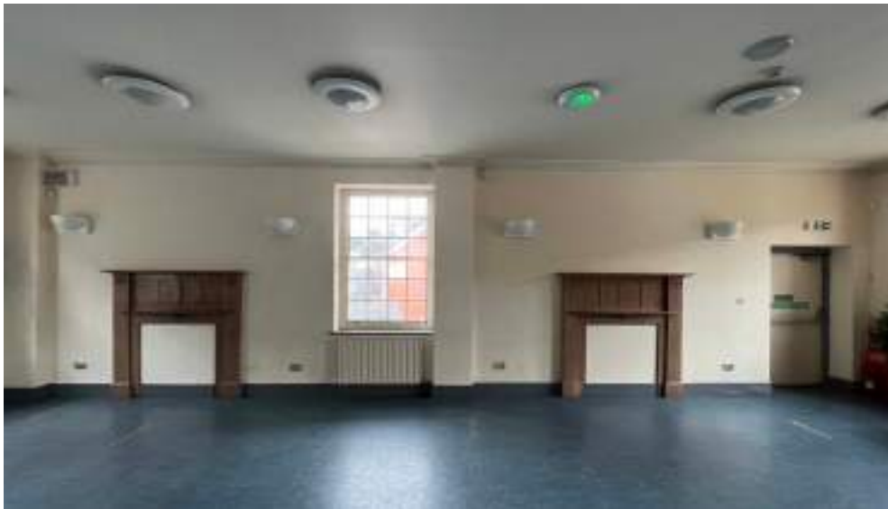
Photograph 95: Timber sash window and original fireplaces
