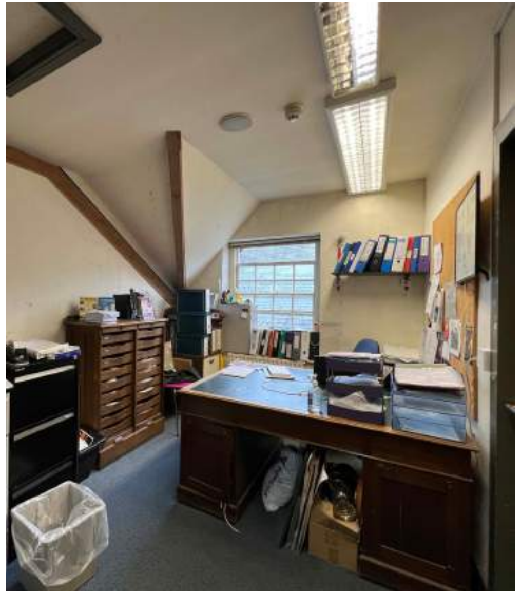
Photograph 104: Timber sash and exposed roof structure
