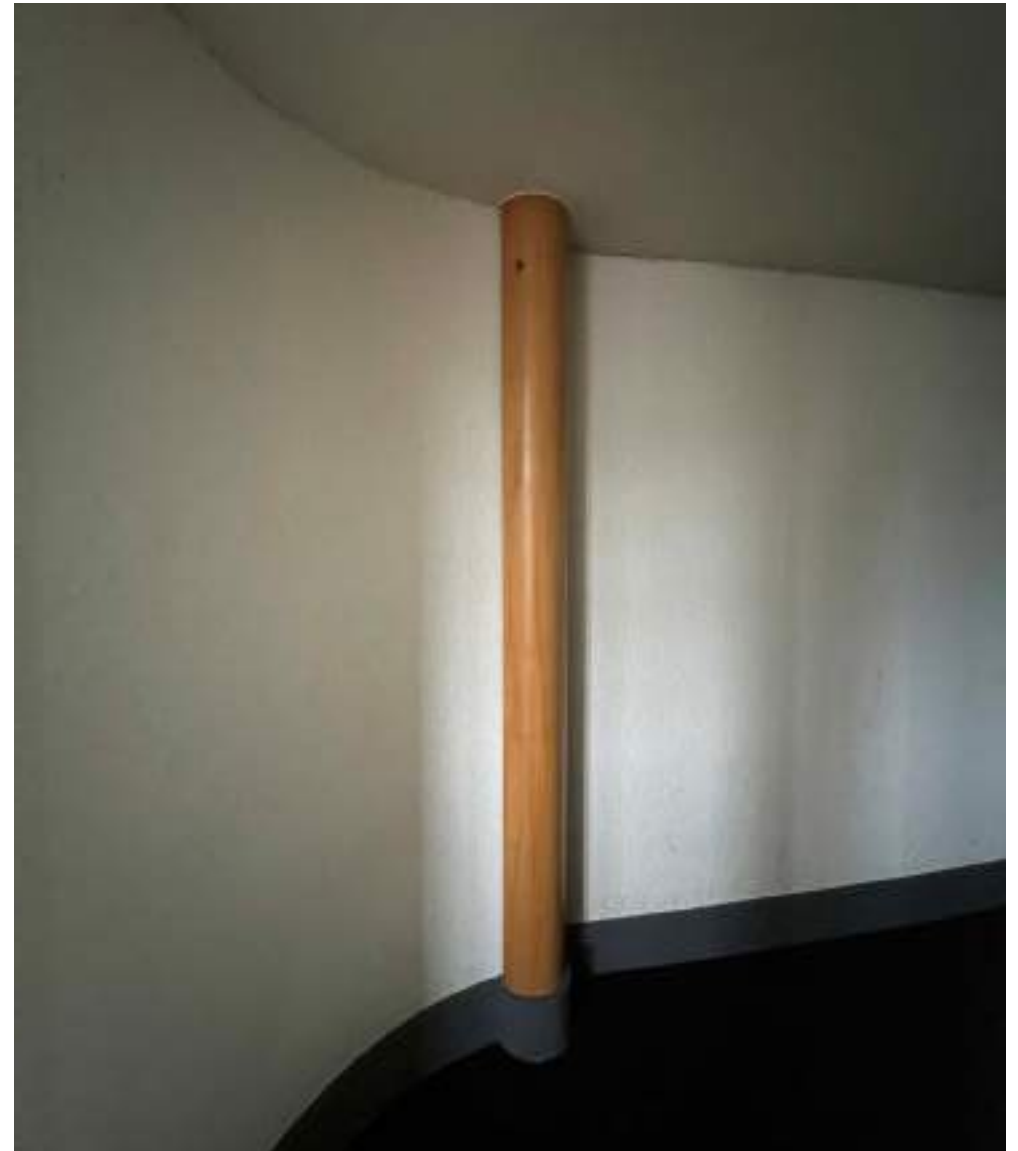
Photograph 83: Modern finishes and veneered timber column casing
