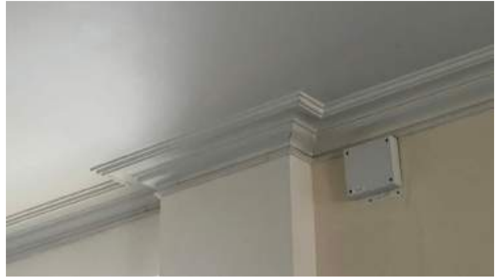
Photograph 94: Original plaster cornice
