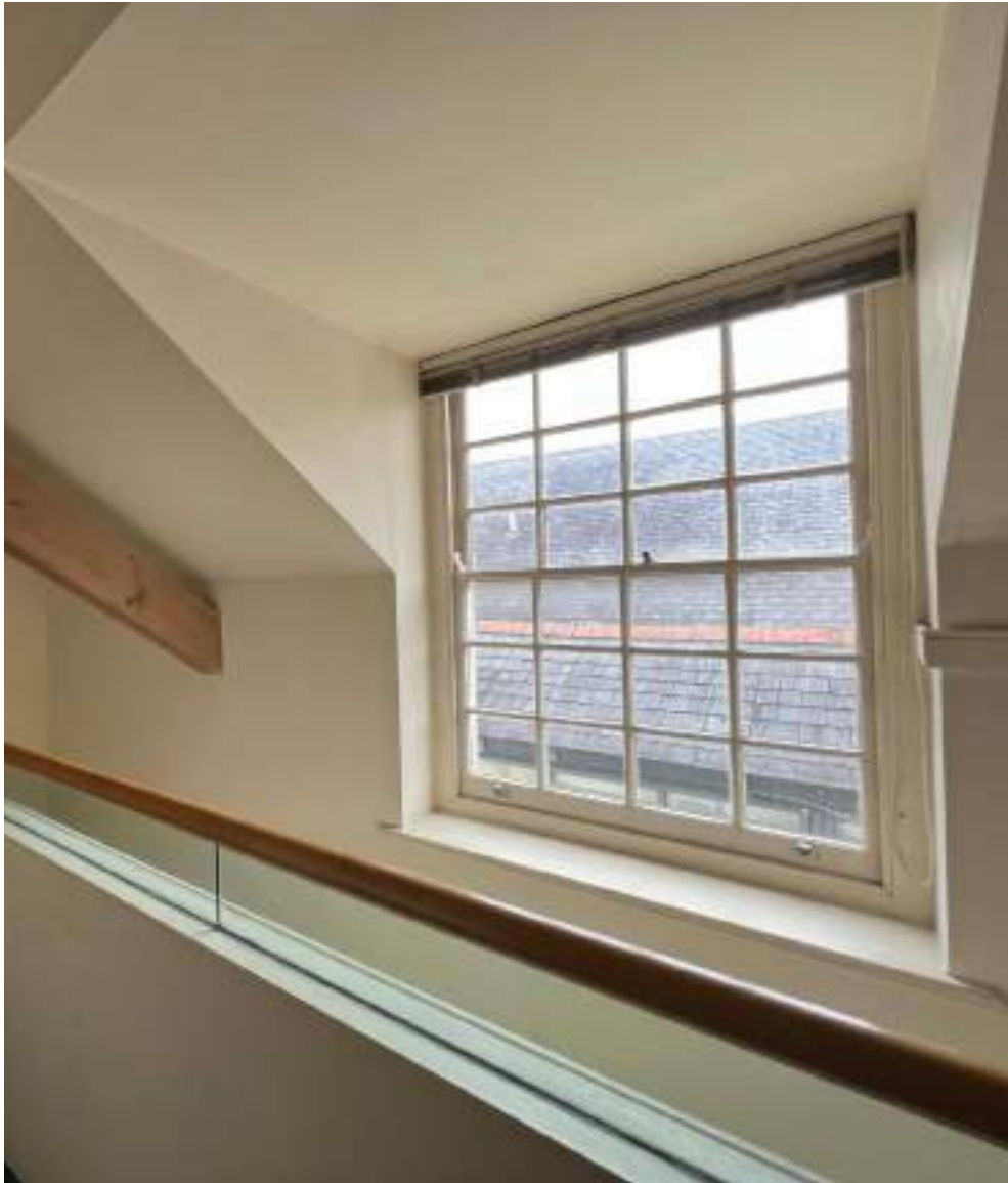
Photograph 102: Original timber sash window
