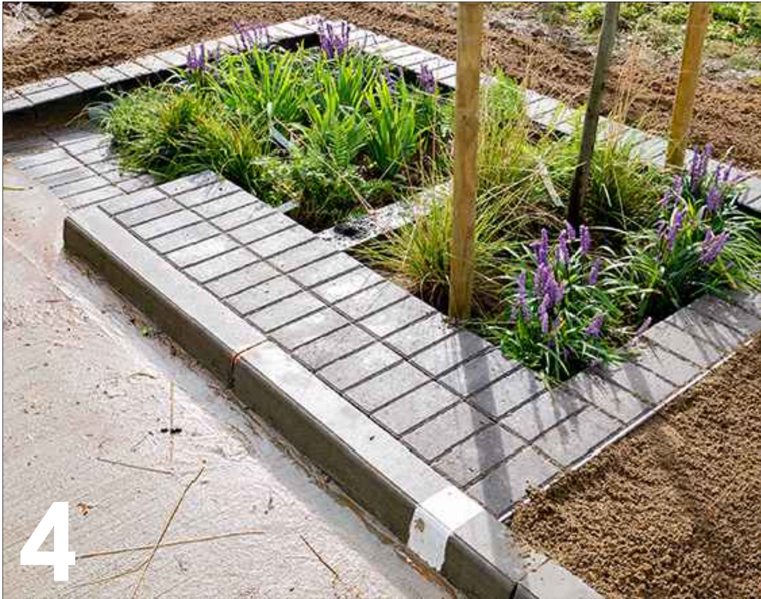
RAIN GARDEN_Hydro planter with drought tolerant planting
