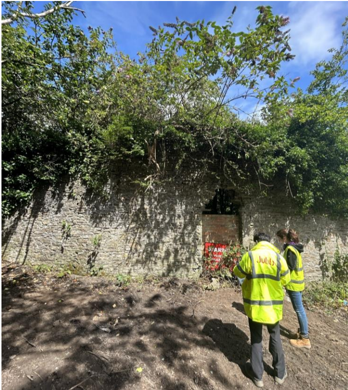
Figure 4.3: Overall extents of the north-west wall (second visit, following removal of some vegetation)
