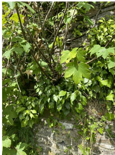
Figure 4.2: Vegetation seen penetrating through the north wall.
