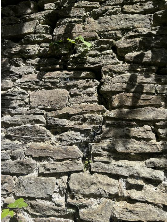
Figure 4.5: Crack seen along the north-west wall.
