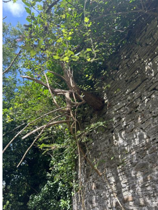
Figure 4.4: Vegetation seen penetrating through the north-west wall.
