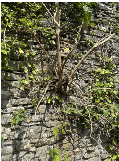
Figure 4.2: Vegetation seen penetrating through the north wall.
