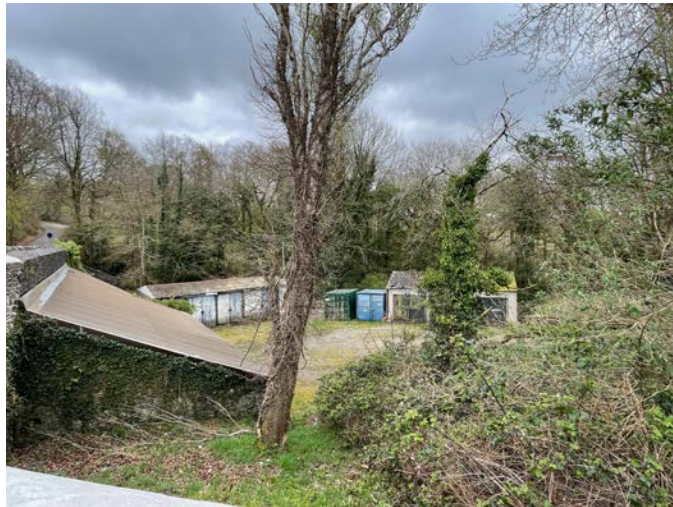
Pump House service yard, looking down from the access road to the east of Pond Cottage
