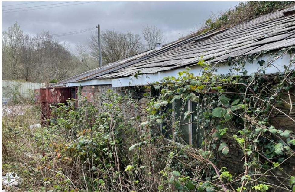
Existing derelict potting sheds - largely stone with brick infill. Overgrown with brambles
