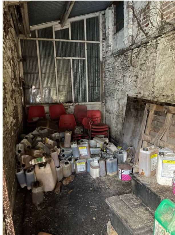
Interior view of the west-facing building showing retaining wall to right and timber frame clad in corrugate sitting atop low masonry wall.
