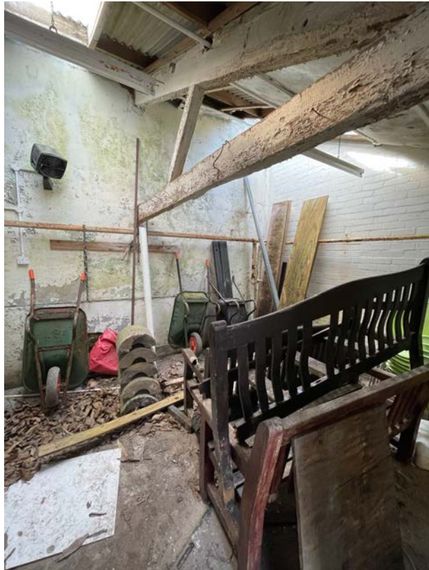
Interior view of the north-facing lean-to potting sheds, showing replacement corrugate roof
