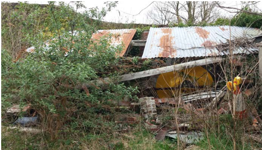
Collapsed glasshouse with later alterations and roof covering -south facing element in area 2
