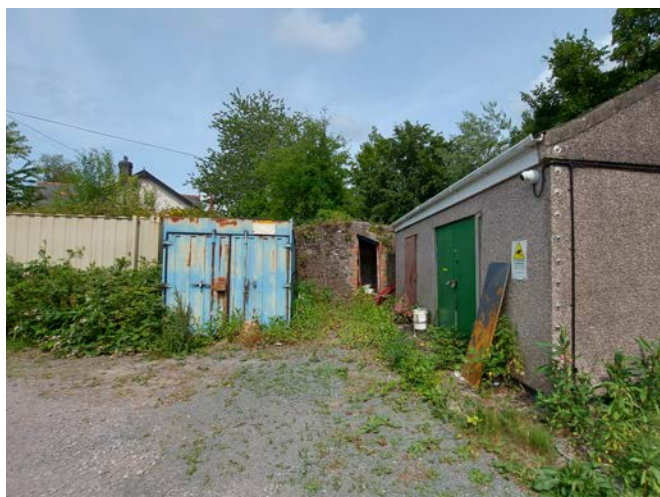
View from Area 3, looking towards the garden wall of Pond Cottage, showing opening into existing WC, containers and existing pebbledash garage.
