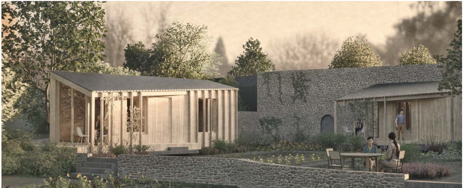
Area 4 - The pods are pre-fabricated and will be delivered to site to sit on pre-laid foundations to suit the levels of the land
