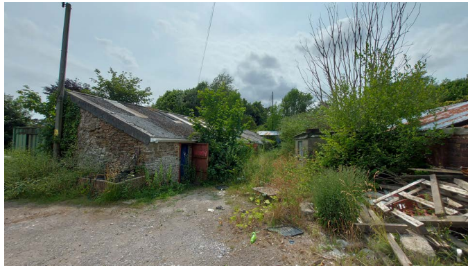
Existing outbuildings, forming a U-shaped group in Area 2
