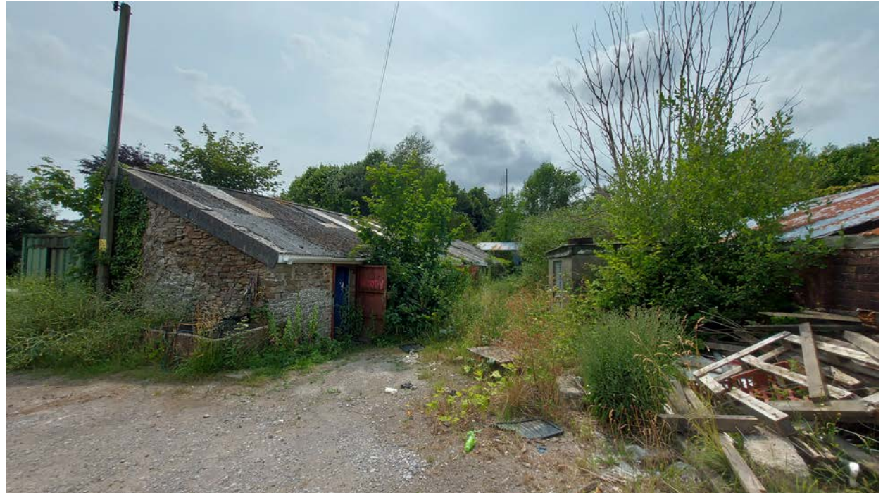
The overgrown derelict, lean-to potting sheds will be taken down
