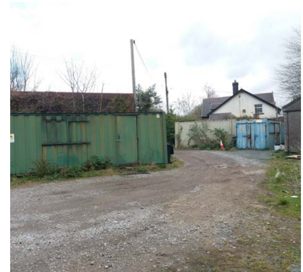
Looking East from the ramped path up to area 4 - short range views of Pond Cottage
