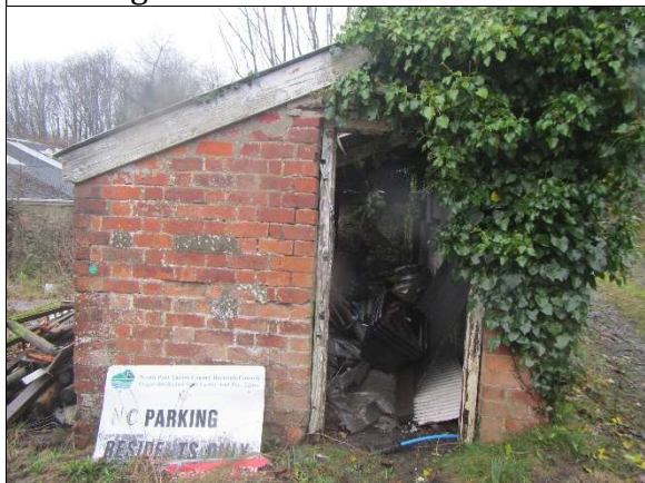
Eastern elevation of northern building
