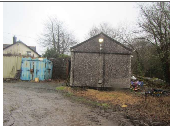
South-western elevation of building in south-east corner of site
