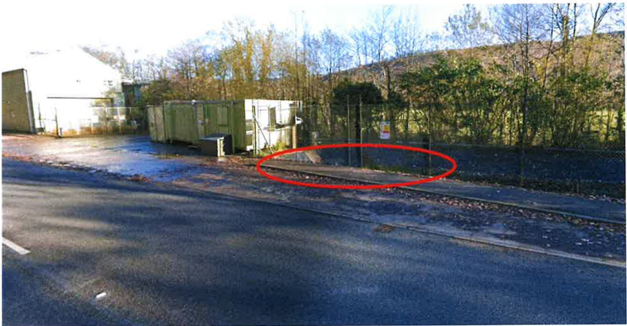
Figure 1 – Existing view identifying the broad location of the highway encroachment
