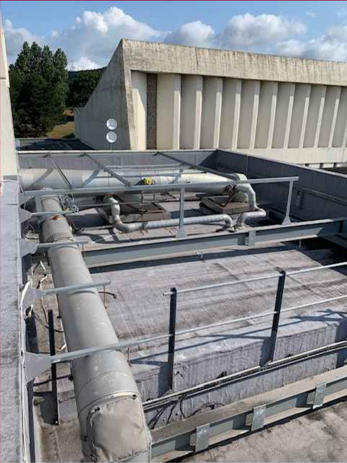
Upper Roof Photograph
