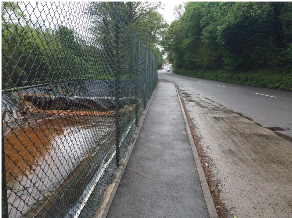
Photograph 4 – View looking south west along the B4242 showing the existing emergency pond feature adjacent to the active treatment plant
