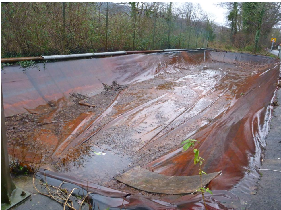
Photograph 5 – The existing emergency pond
