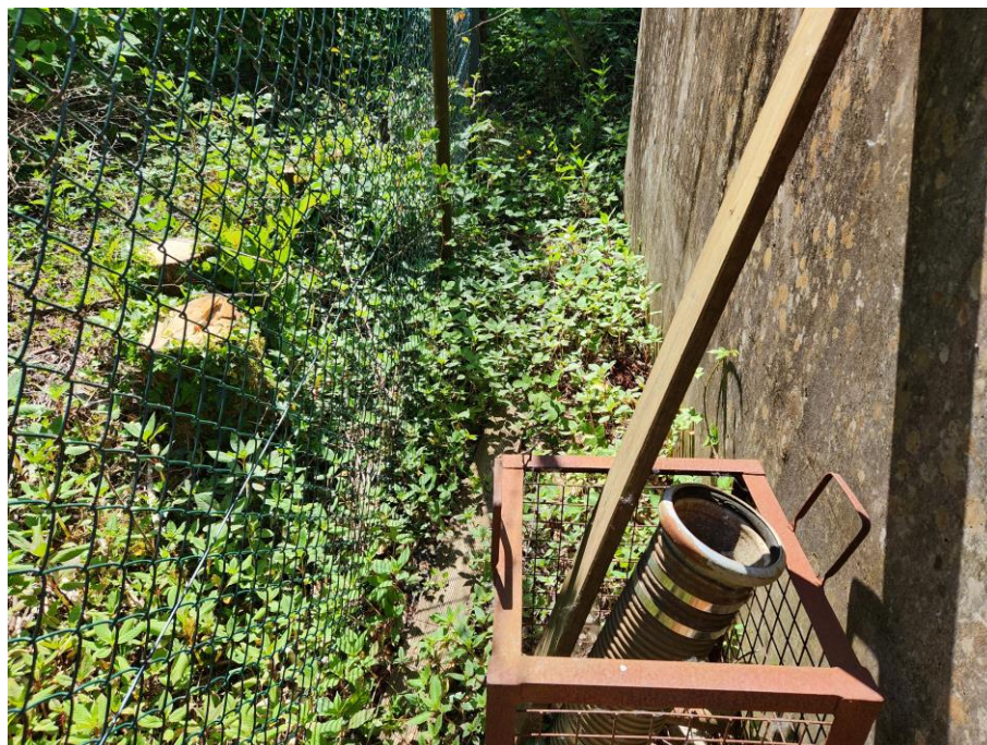
Figure 6: Himalayan Balsam growing along NE boundary.
