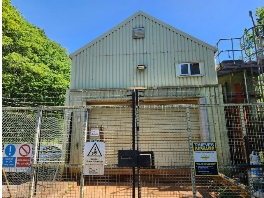
Figure 5: SW façade of current treatment building.
