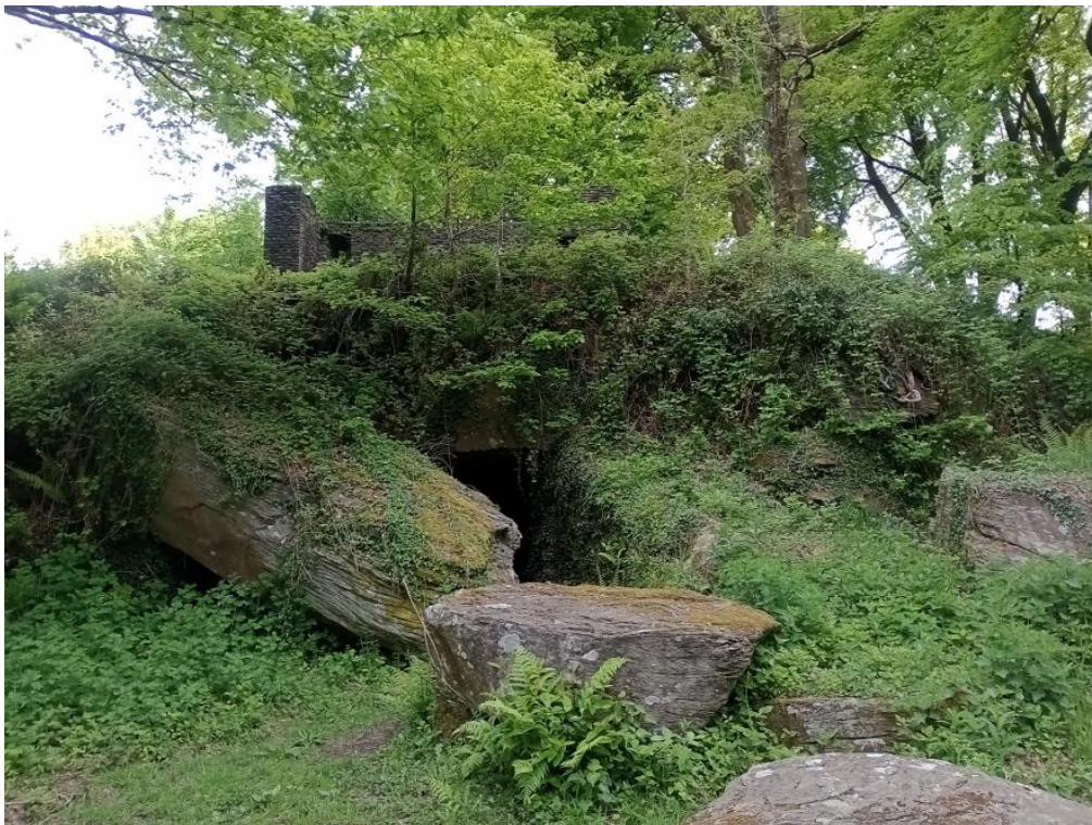
Photo 34: View east of the entrance to the grotto with the remains of a structure above (PRN 01948w/07364w).
