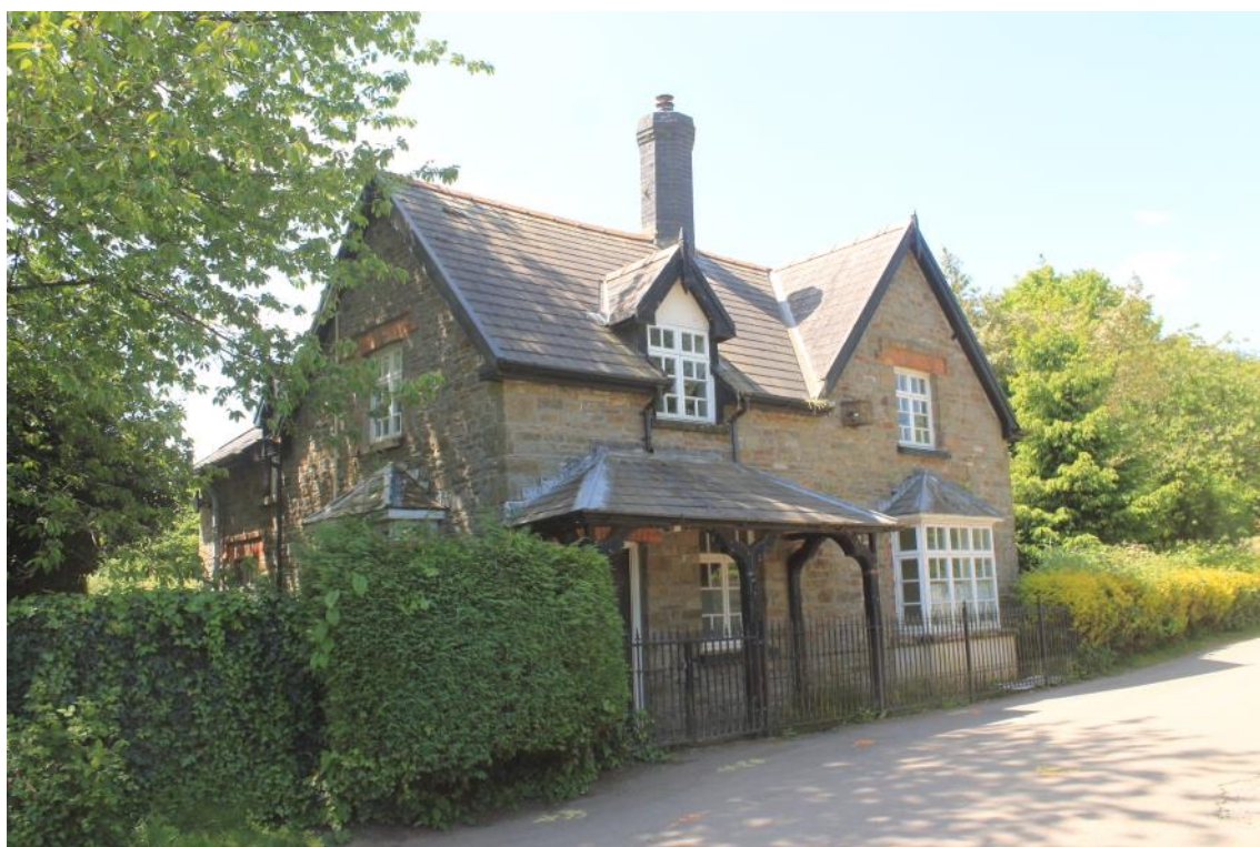
Photo 20: View southwest of Pond Cottage GP37.
