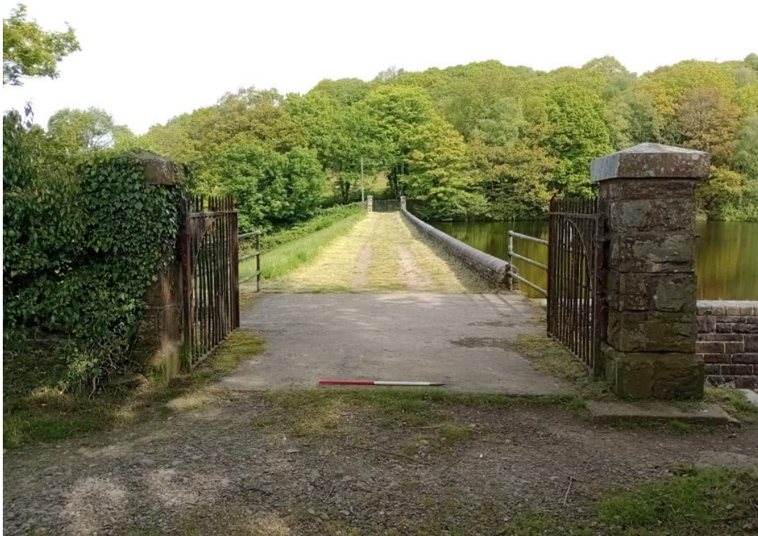
Photo 29: View south of the gate entrance to the north part of the estate across the Mosshouse Woods Reservoir (PRN 06094w) bridge/dam. 1m scale.
