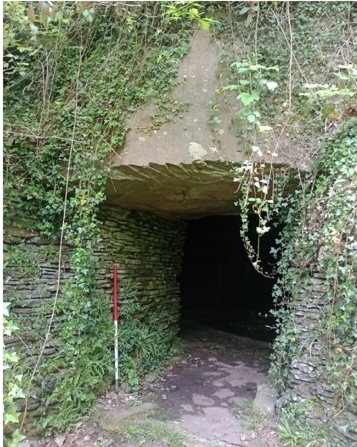
Photo 33: View northeast of the entrance to the grotto PRN 01948w/07364w. 1m scale.
