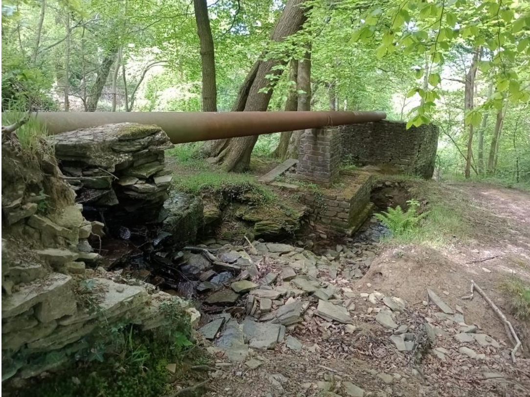
Photo 30: View southwest of structure PRN 07365w at the head of the informal cascades LB 22870.
