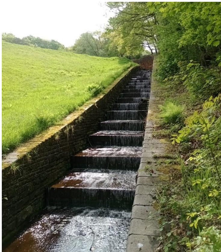
Photo 28: View southeast up the overflow for Mosshouse Woods Reservoir PRN 06094w.
