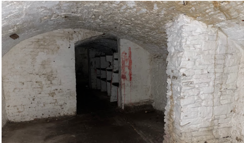
Interior view of the cellar showing lime washed finishes. The structure is in a reasonable condition generally
