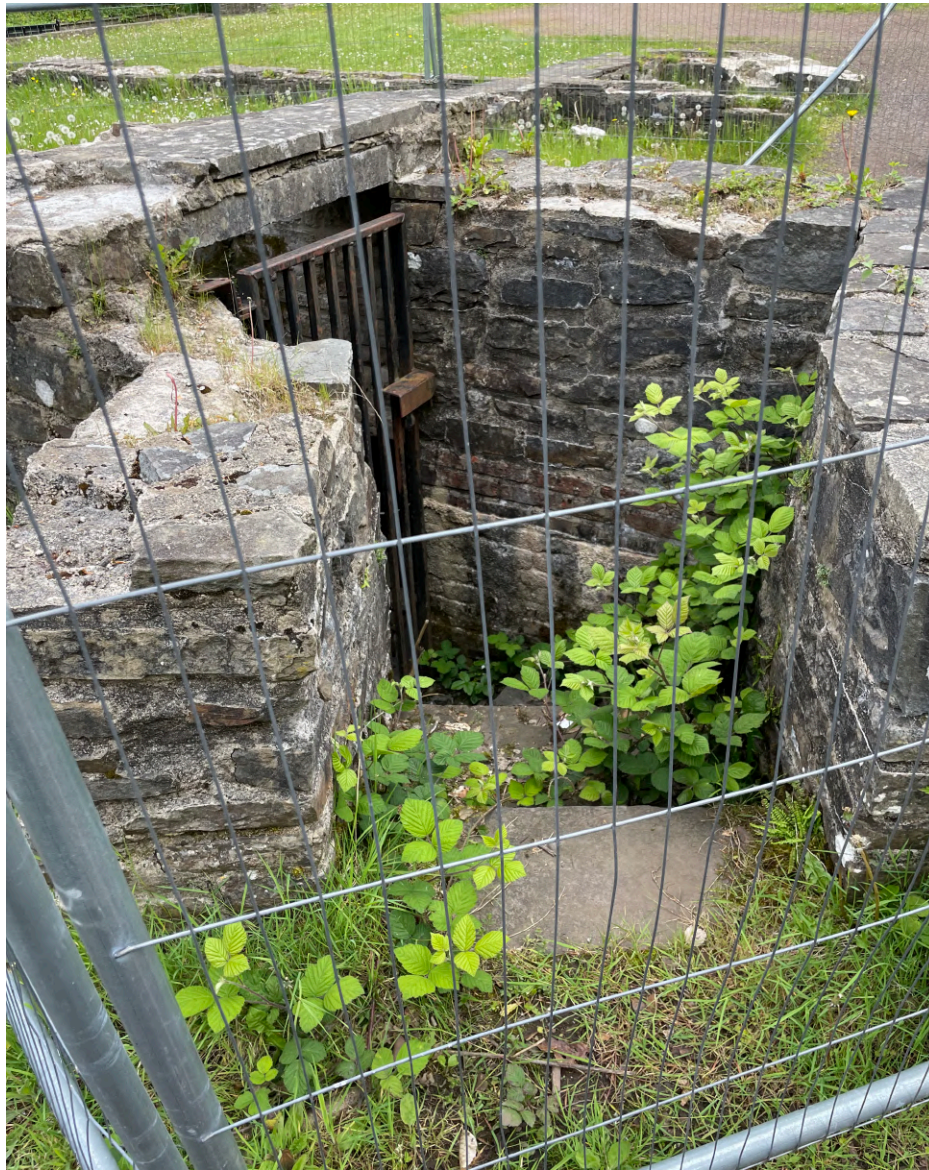
Existing stonework will be consolidated as part of the proposed repairs
