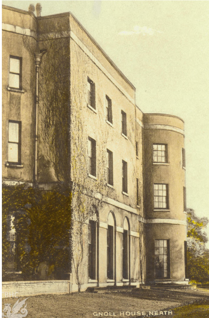
The house following the removal of the North West wing. This undermined the formal frontage.
