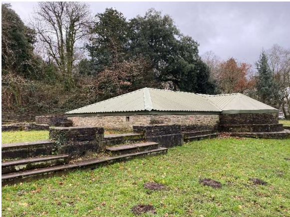
Stone-built building with corrugated roof (north & western elevations)
