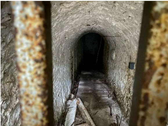
Internal view of north-western entrance
