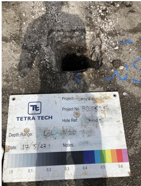
Plate 13 WS05 inspection pit following excavation to 1.20m bgl.
