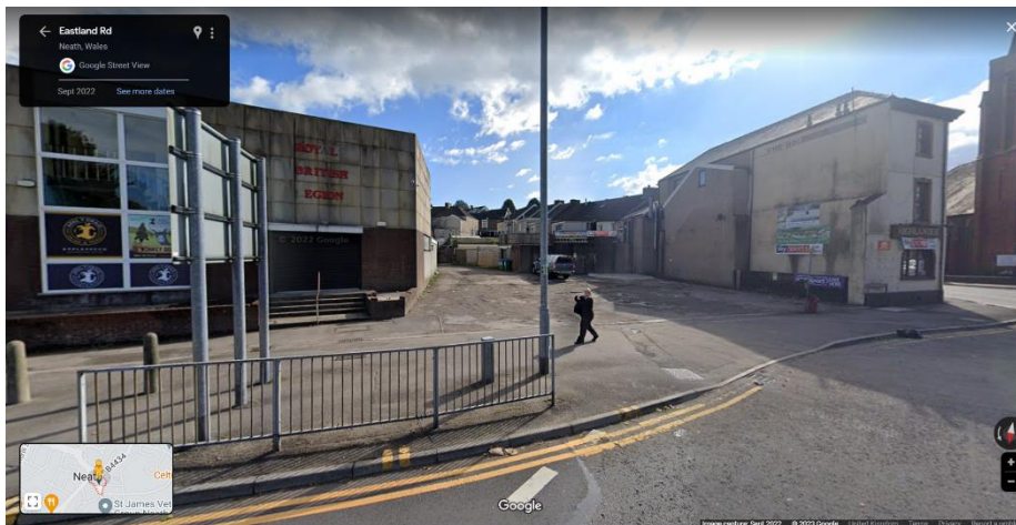
Figure 3. Car park access from the southern approach (Google Maps, September 2022).
