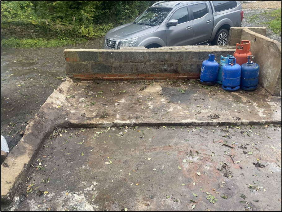
Pic.6 View of slab / perimeter toward South West.
