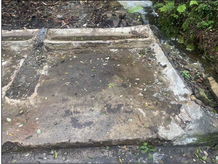
Pic.5 Concrete floor slab - remnants of division panels and feeding trough along the rear wall base.
