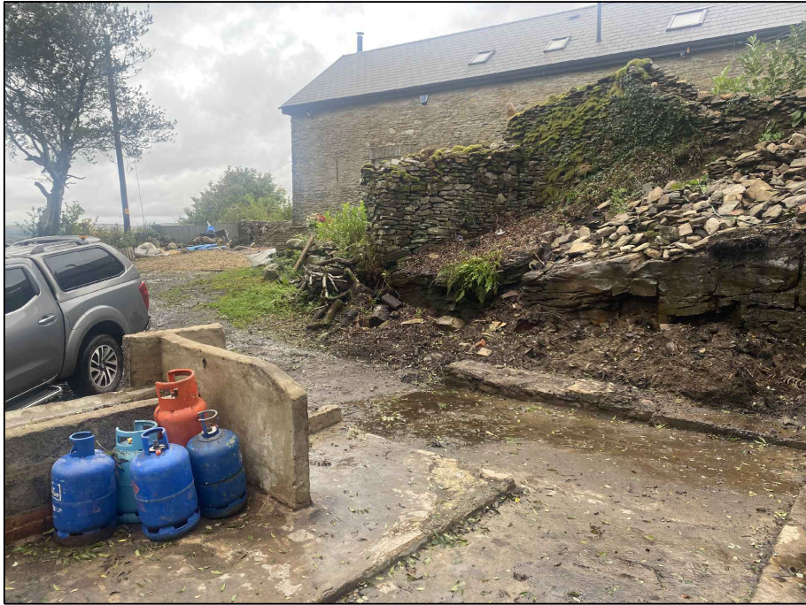
Pic.7 View of slab / perimeter toward North West (vehicle entrance point).
