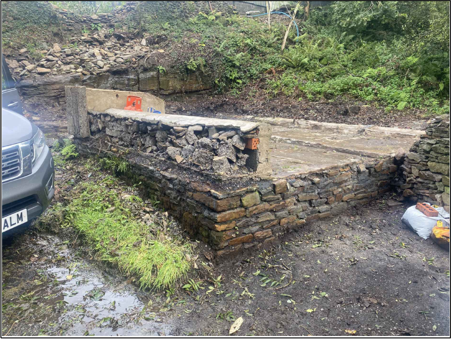
Pic.4 The remaining substructure walls viewed from the South West aspect - natural stone walling used to form the perimeter along the sloping site. A small section of concrete block wall was present to the front elevation only
