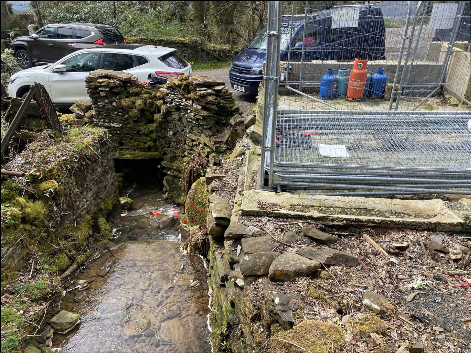
Pic.18 View of stream adjacent to edge of barn slab. Note close proximity of the slab to the stream - this was intentional at the time of original building - as there is a wash out channel from the barn (milking shed) to directly into the stream - for the disposal of cattle waste. The dry stone walls that form the side of the stream bank and the above ground section preventing fall into the stream are in poor condition and will likely need taking down and rebuilding due both due to the likelihood of disturbance during the works and the obstruction of some elements.
