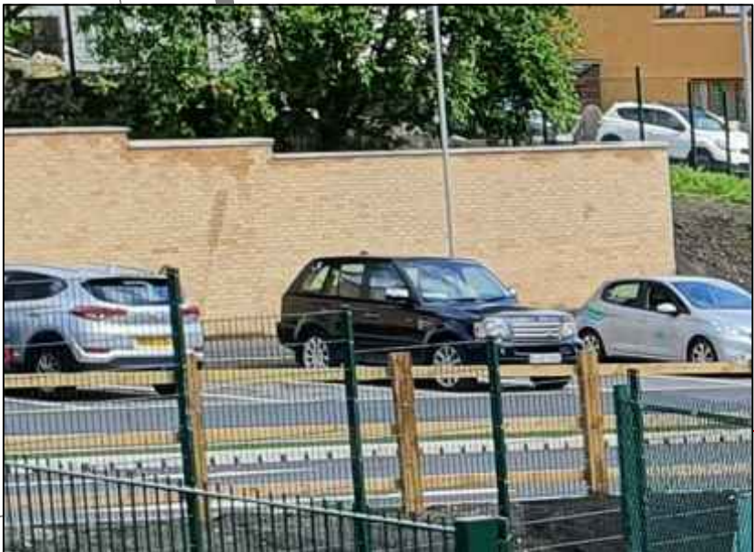
EXISTING SCHOOL RETAINING WALL
