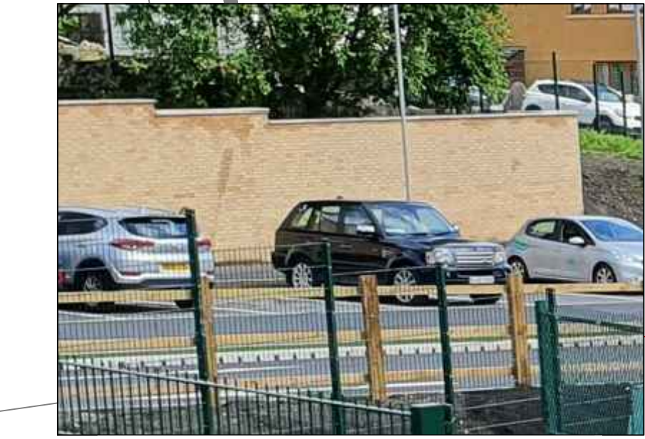
EXISTING SCHOOL RETAINING WALL
