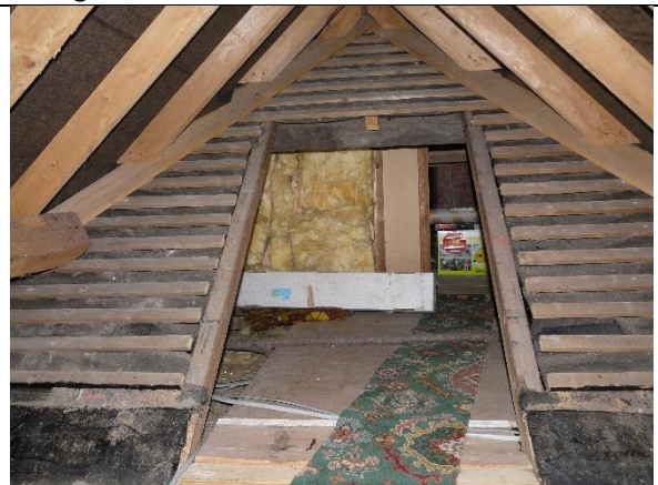
Photo 22: Internal view of loft spaces
