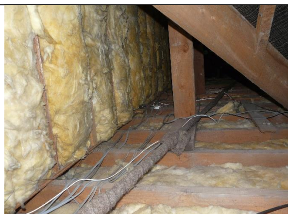
Photo 26: Internal view of eaves loft spaces
