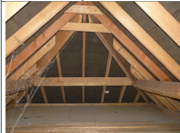
Photo 21: Internal view of loft spaces
