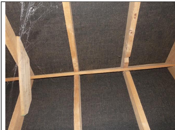
Photo 19: The concrete tile roof is lined with black bitumen roofing felt
