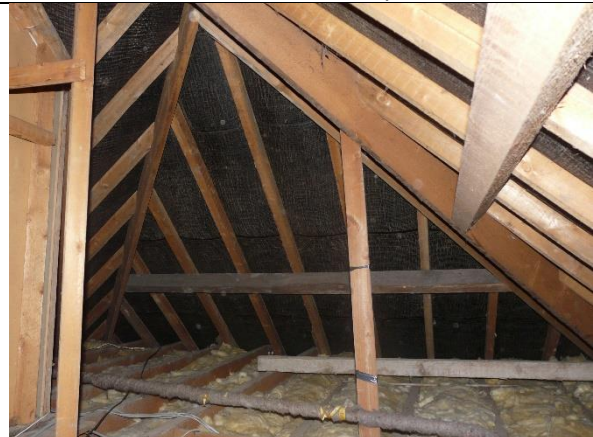
Photo 24: Internal view of loft spaces
