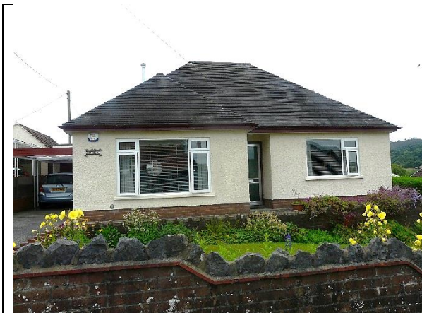
Photo 1: North facing front
