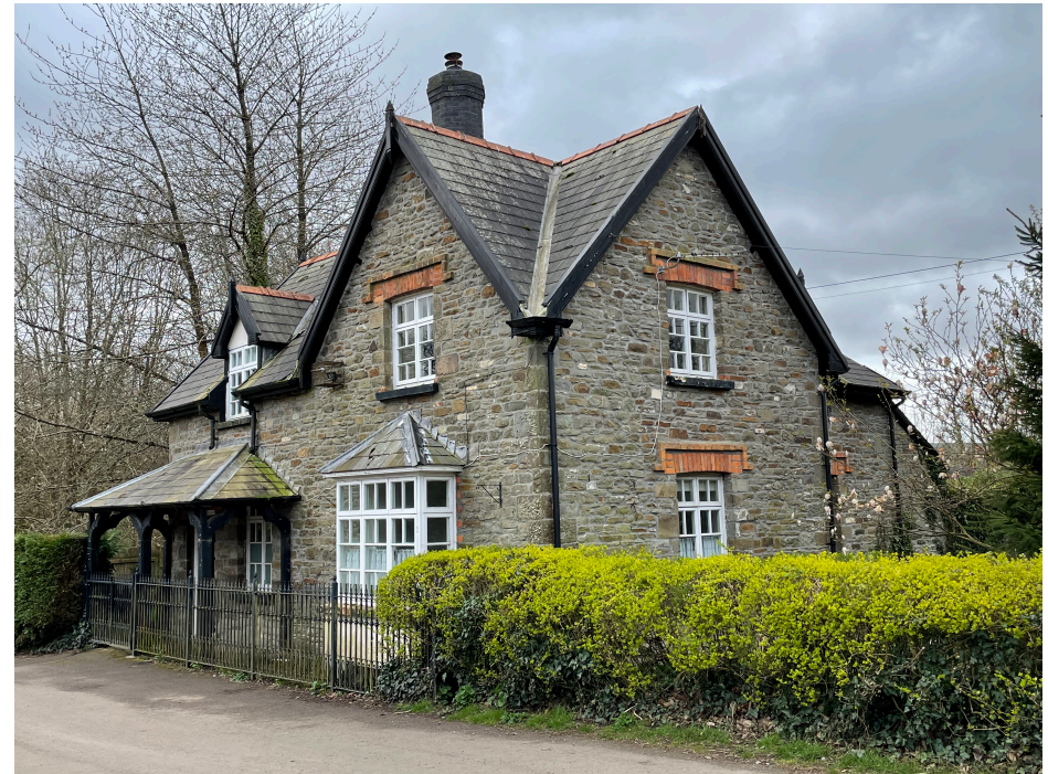
Access into the ground at Pond Cottage is predominantly via the railings to the frontage. This borders the principal pathway that loops around the fishpond
