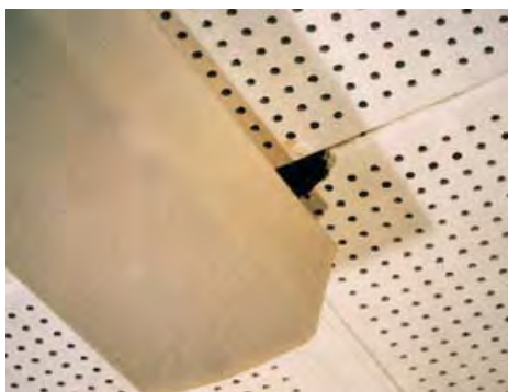
Figure 6 Perforated AIB ceiling tiles
