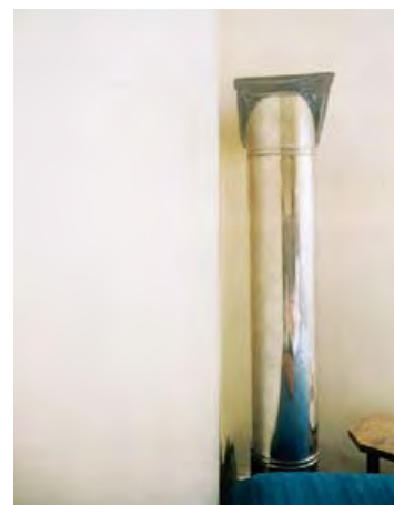
Figure 11 Metal/asbestos flue pipe – the asbestos is between the inner and outer layers of stainless steel
