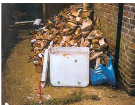
Figure 12 Asbestos cement tank
