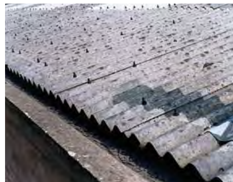
Figure 7 Asbestos cement roof
