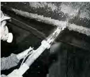
Figure 36 Installing a sprayed 'limpet' coating
