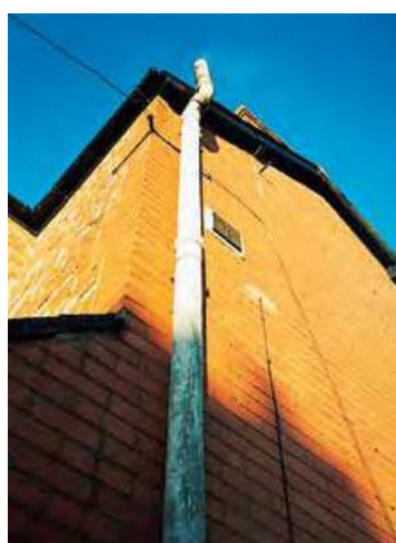
Figure 17 Asbestos cement flue – external
