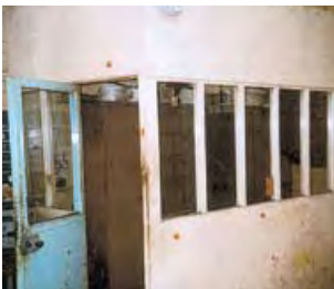
Figure 28 An office made from AIB
