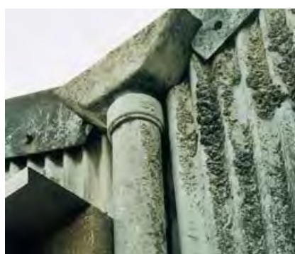
Figure 15 Asbestos cement drainpipe
