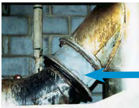
Figure 10 Flexible asbestos duct connector (gaiter)
