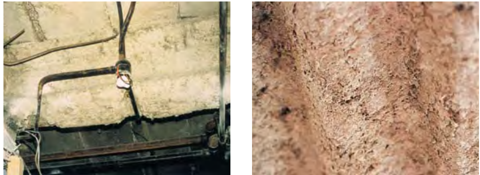
Figure 30 Distance (left) and close up (right) pictures of sprayed 'limpet' asbestos coatings. These can contain up to 85% asbestos which is loosely bound. This type of material readily releases fibres when disturbed
