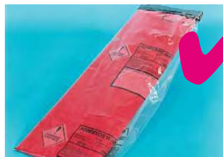
Figure 57 Door with an AIB panel wrapped in polythene sheeting
