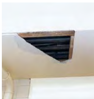
Figure 40 Damaged AIB
