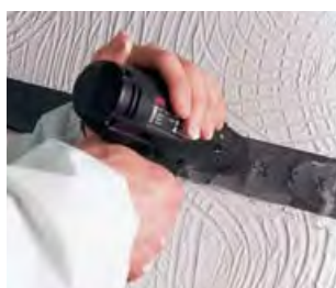
Figure 50 Drilling through paste
