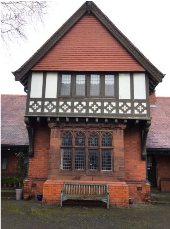
General view of central range's S elevation, showing 1st floor's exposed jettied timber frame
