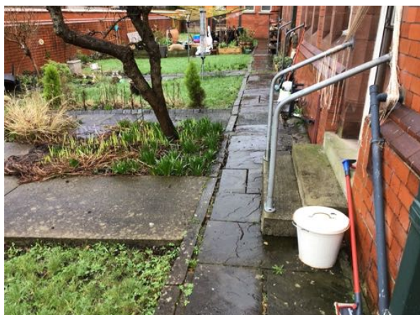
W rear path, viewed from W end
