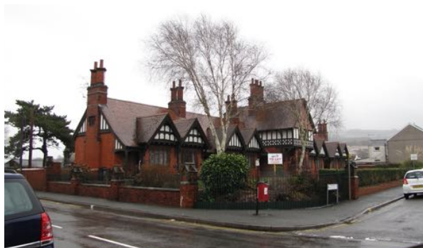
View of Llewellyn Almshouses from SW (Gnoll Park Road)
