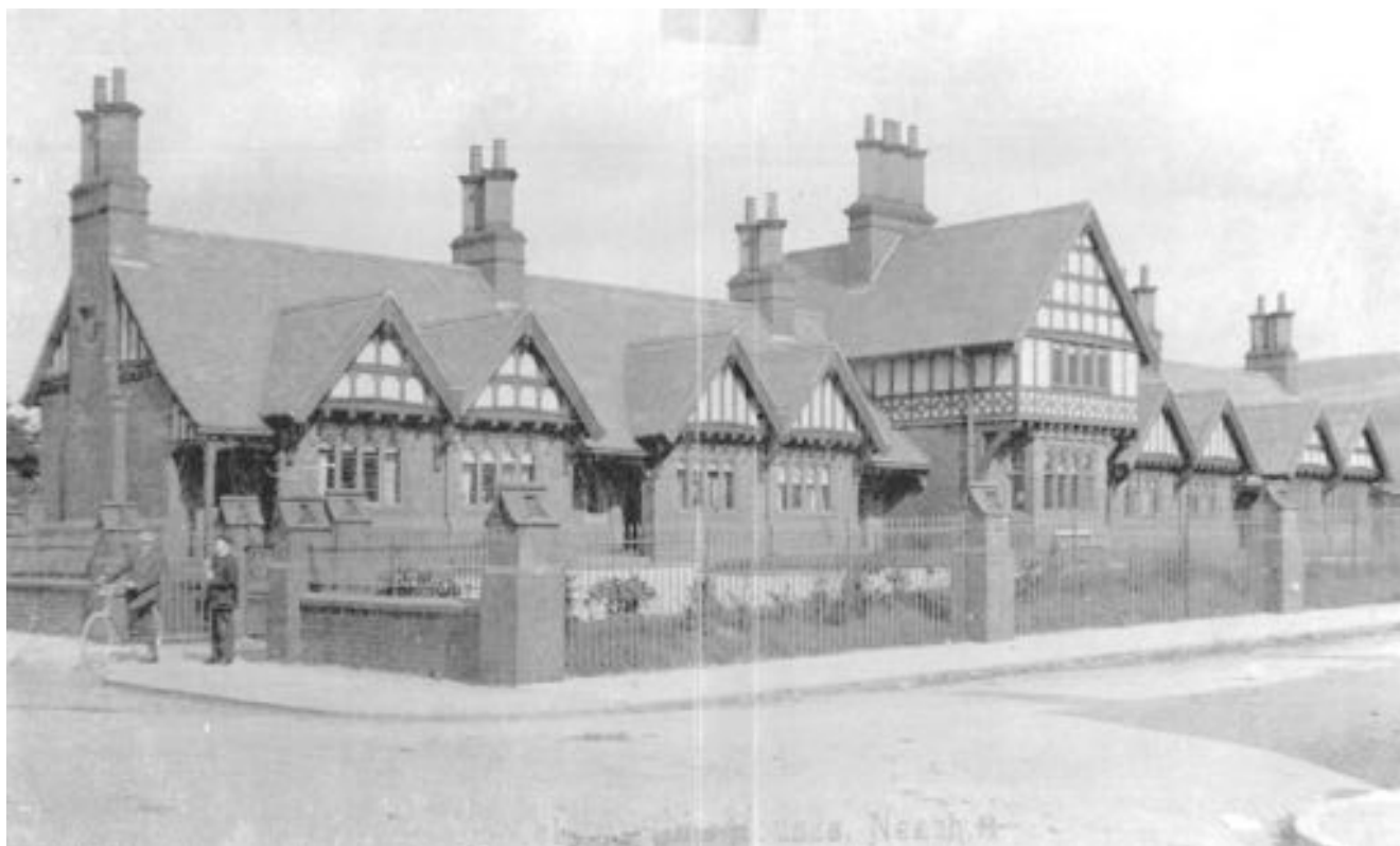
Historic photograph of Llewellyn Almshouses shortly after it was built
