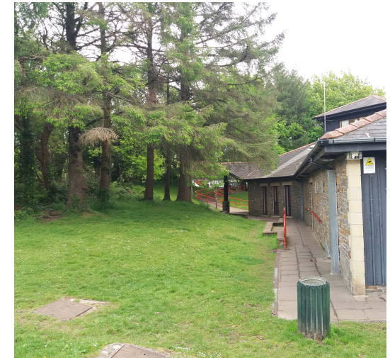
North façade of existing building, with tree-lined slope behind
