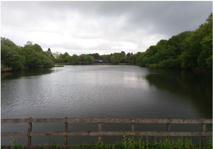
View from the dam to the south of Fish Pond
