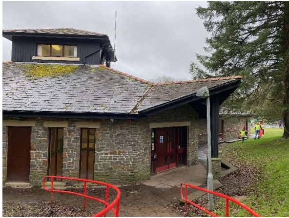
North-eastern and portion of north-western elevations.
