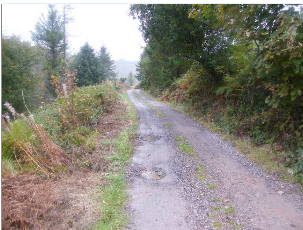
Photo 2: Fforch-Dwm Road inside scheduled area (GM458), looking north-west
