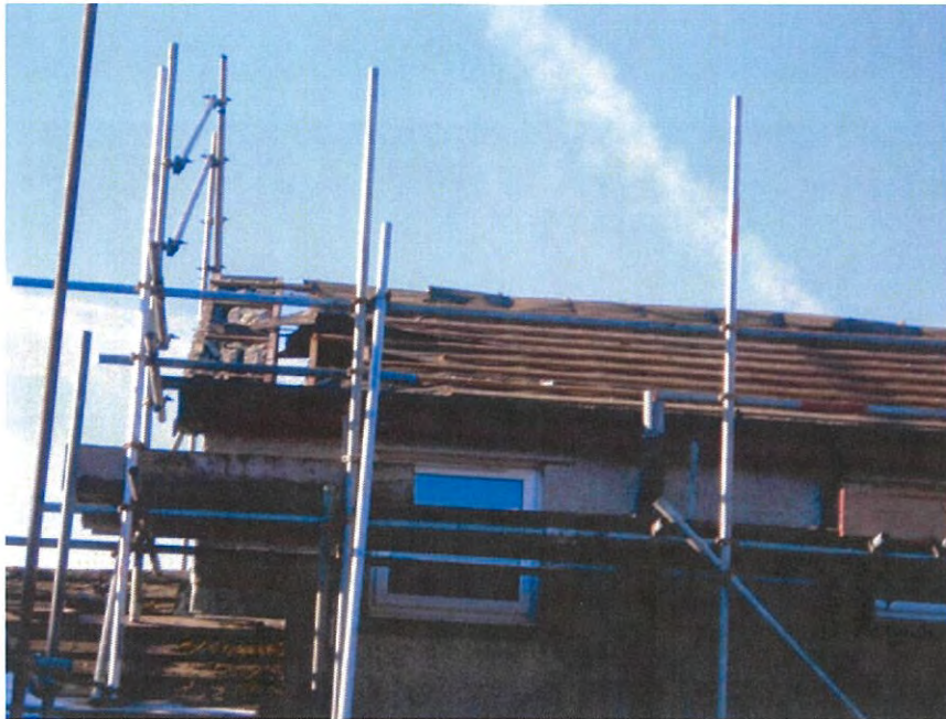
Work on the caretaker's house
