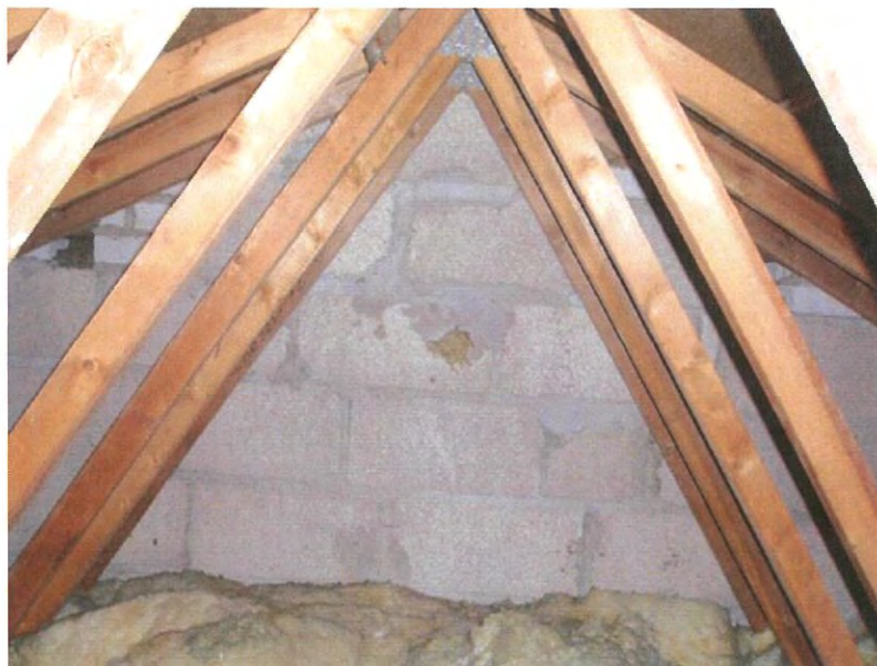
Typical roof structure
