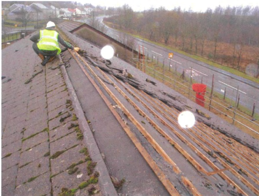
Work on the eastern section roof
