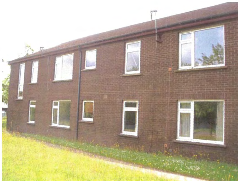
The Eastern Wing, northern elevation
