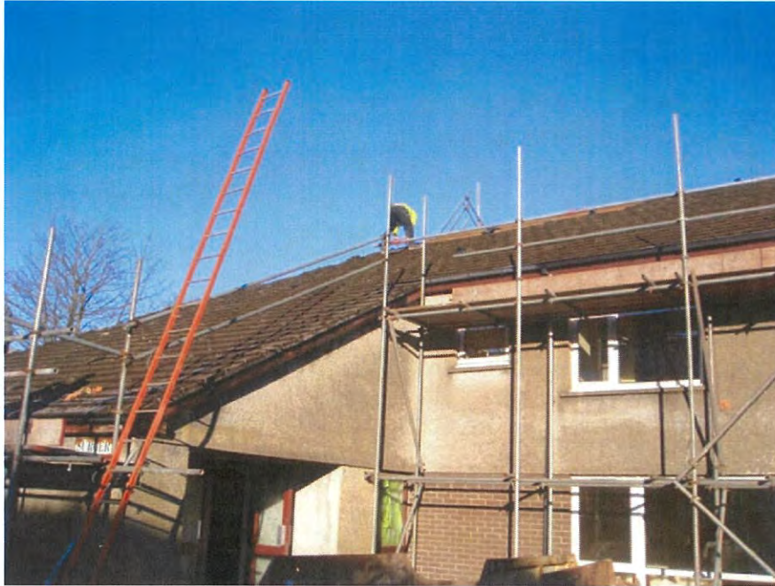
Work starting on the western section 2015
