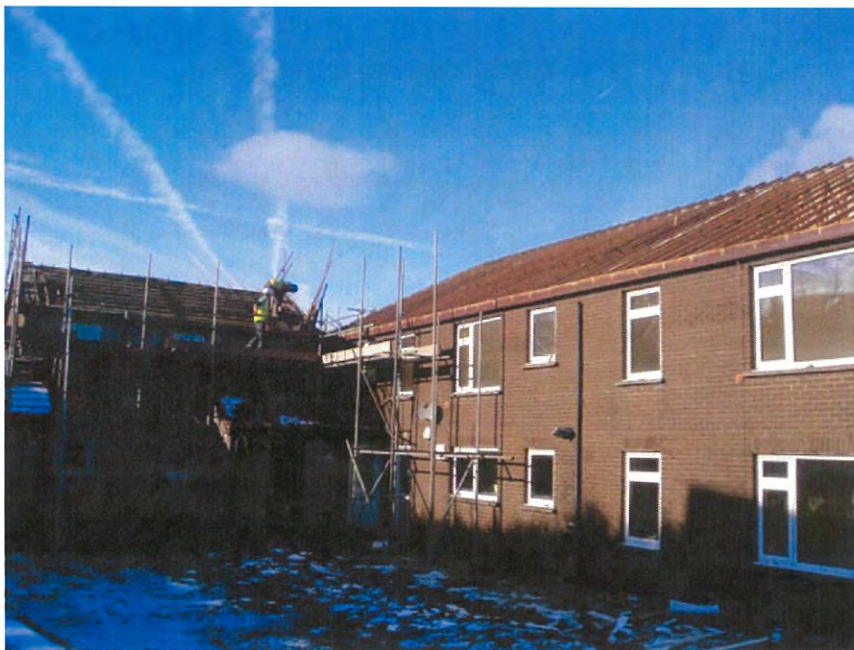
The caretakers House and the stripped eastern section
