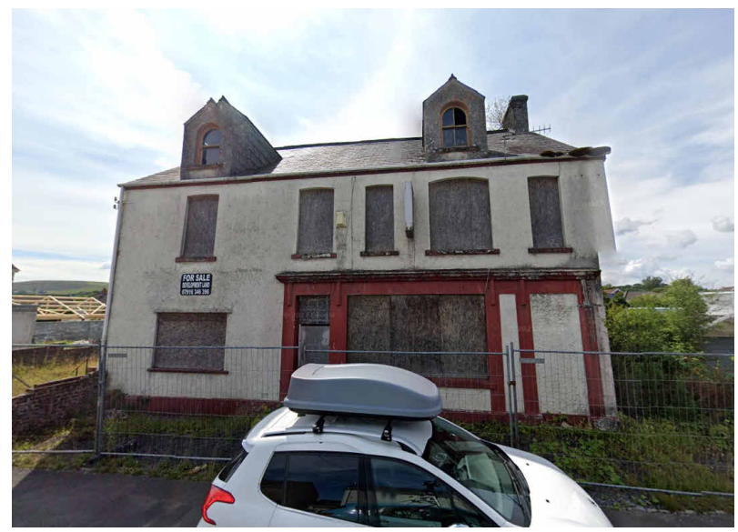
Existing building on site to be demolished.
