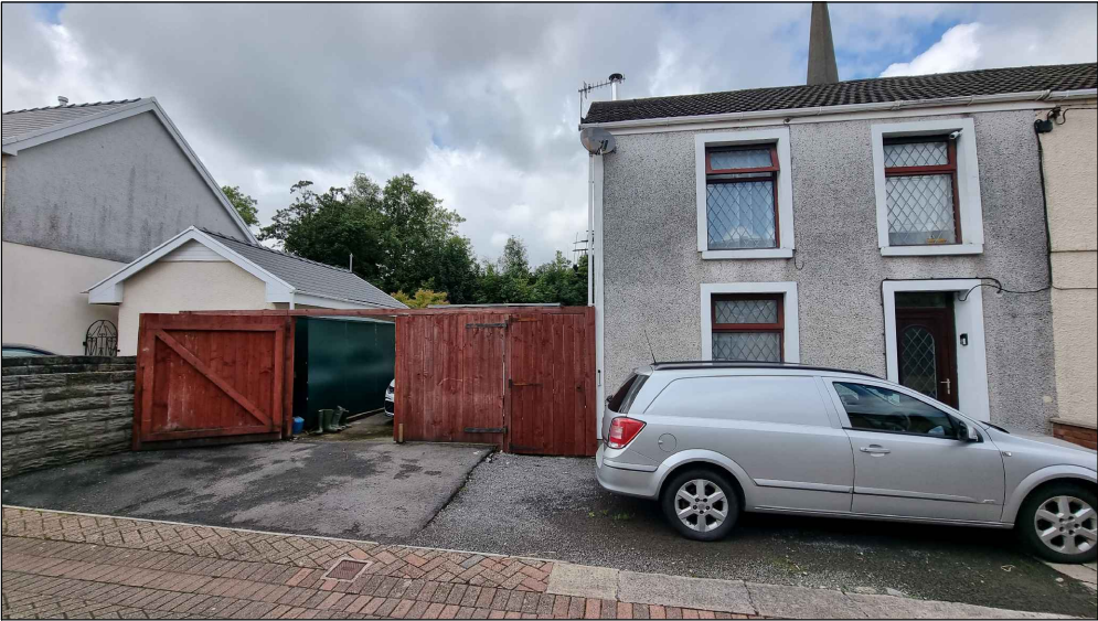
Site Photograph indicating existing street scene
