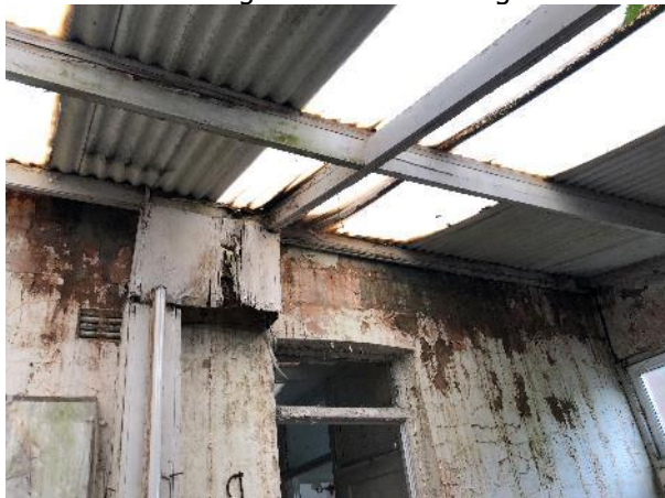
Photo 3: B1 Corrugated Plastic Roofing
