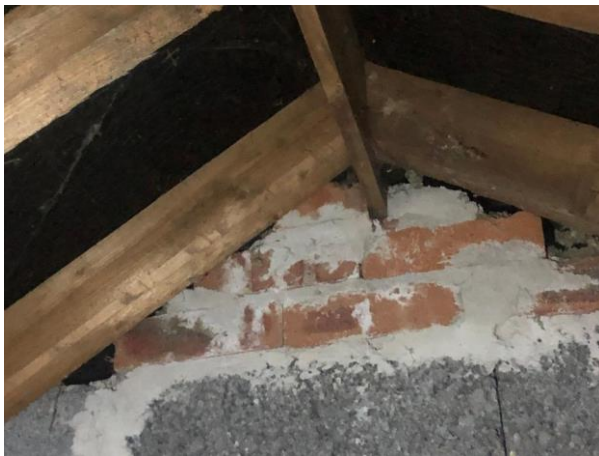
Photo 21: B2 Bitumen Felt Roof Lining
