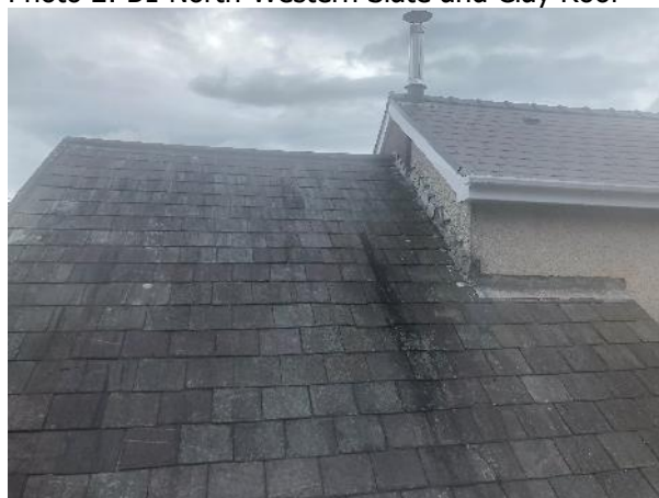
Photo 4: B1 Lifted Slate and Clay Ridge Tile
