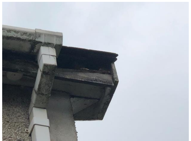
Photo 16: B2 Missing Soffit/Fascia
