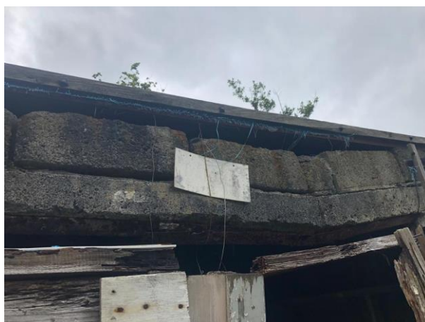
Photo 28: Gaps Between Roofing and Walls
