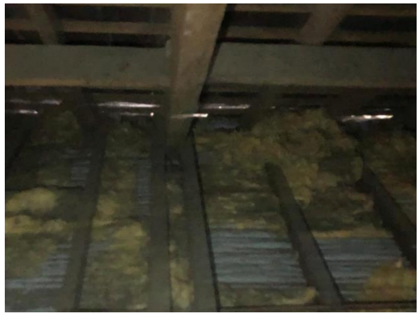
Photo 22: B2 Fiberglass Insulation in Voids
