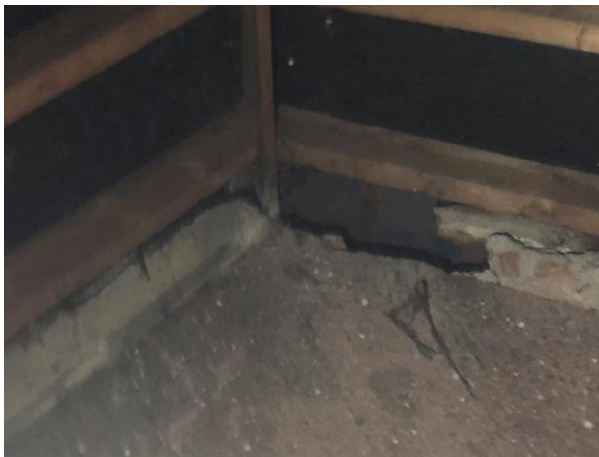
Photo 21: B2 Bitumen Felt Roof Lining
