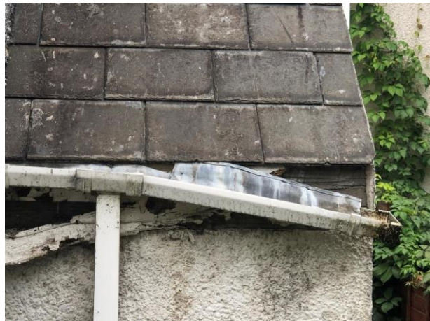
Photo 16: B2 Missing Soffit/Fascia
