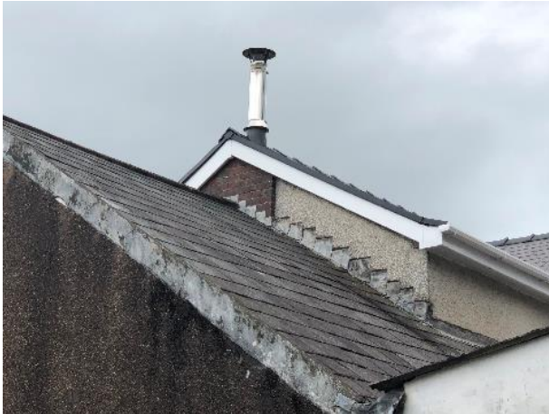
Photo 7: B1 Lead Flashing Around Dormer Window
