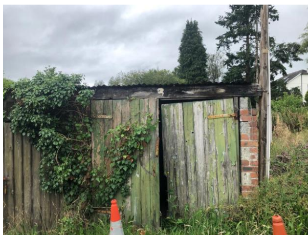
Photo 28: Gaps Between Roofing and Walls
