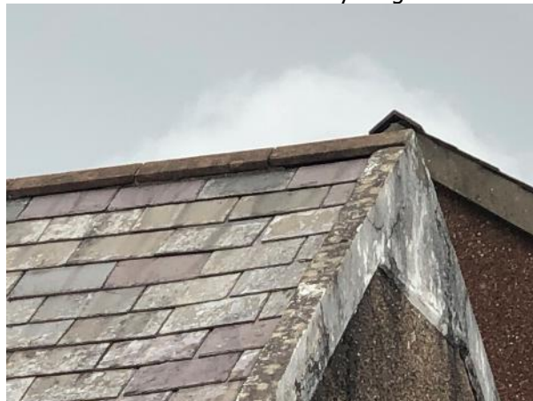
Photo 4: B1 Lifted Slate and Clay Ridge Tile
