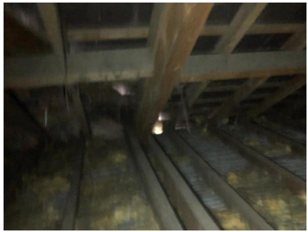
Photo 22: B2 Fiberglass Insulation in Voids
