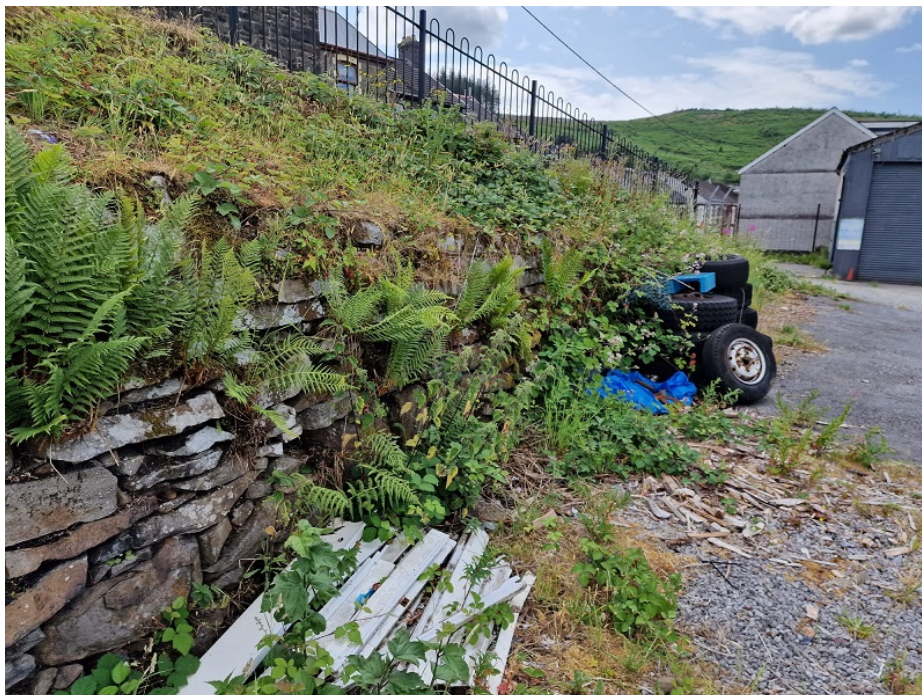
View of lower section of wall
