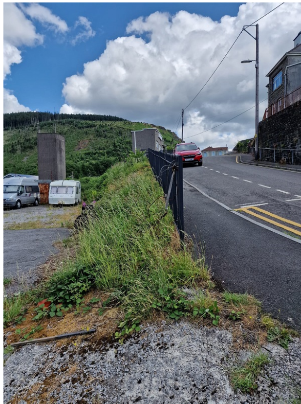
View of footpath to rear of wall
