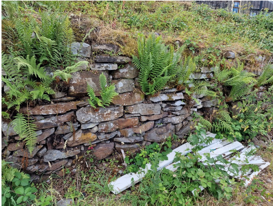
View of wall construction
