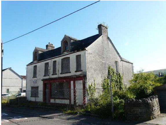
Image 2: Front (east) and north elevations of building
