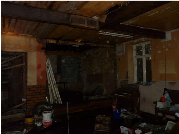
Image 8: Ground floor of building - northern area
