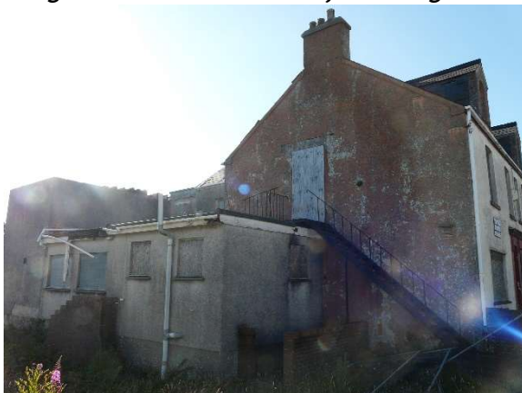
Image 3: South elevation of building
