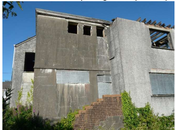
Image 6: Rear (west) elevations - numerous window openings and open roof
