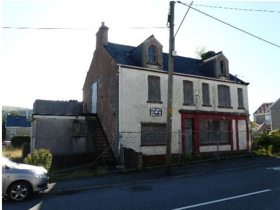
Image 1: Front (east) and south facing elevations of building
