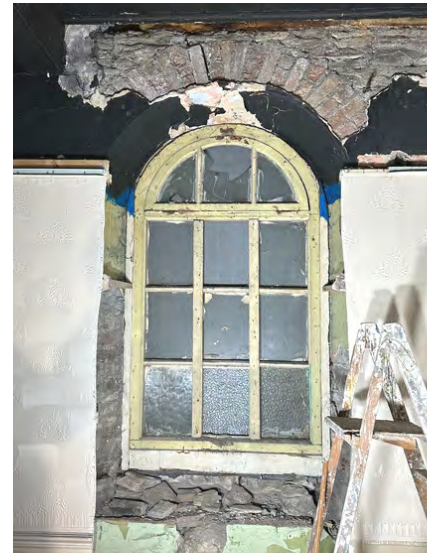
Fig 36: Removal of plasterboard in social room reveals contemporary single glazed timber window
