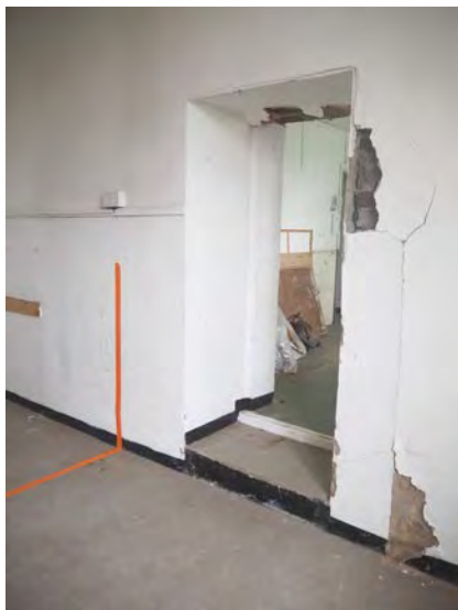
Fig 33: Access between kitchen and kitchen store through unsupported doorway.
