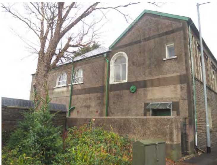
Fig 7: Former Wesleyan chapel structure with hipped slate roof to the northern part of the site (LHS of photograph) and later, gabled structure to the south and fronting onto Castle Street (RHS of photograph).
