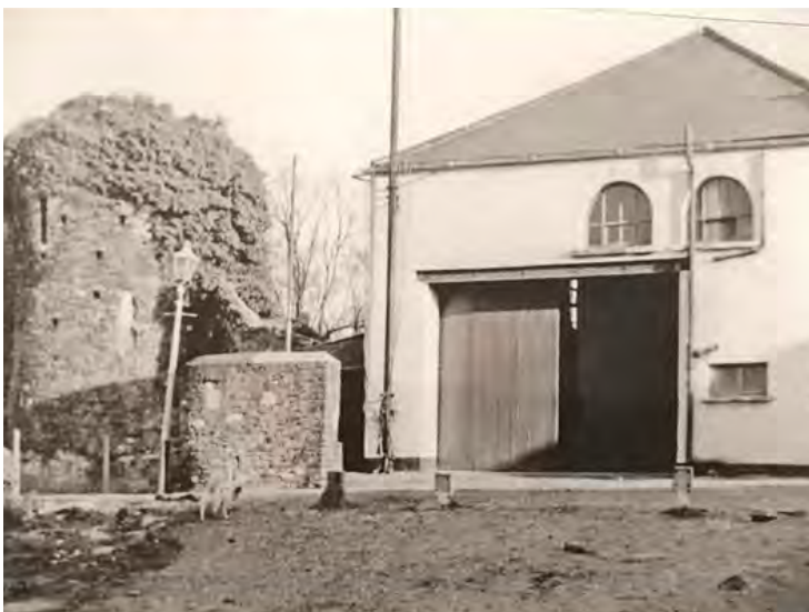
Fig 52: The west elevation of the former chapel transformed to accommodate a fire appliance inside the building. The side road, providing vehicular access to the building remains. Due to the decline in appearance shown in later photographs (see below), it is believed that this image was taken early in the buildings tenure as Neath Fire Station.
