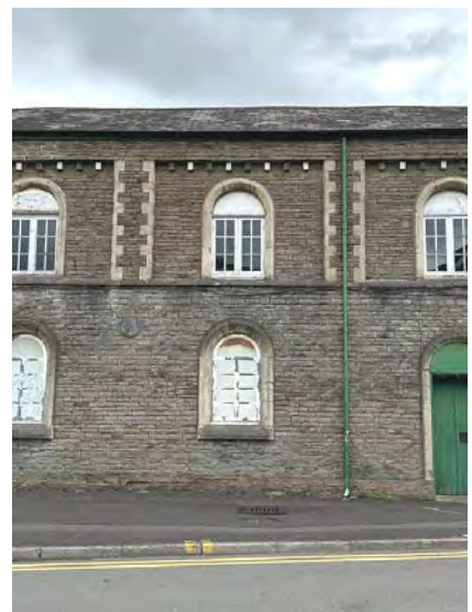
Fig 8: More decorative south elevation incorporating bath stone detailing and window surrounds facing onto Castle Street.
