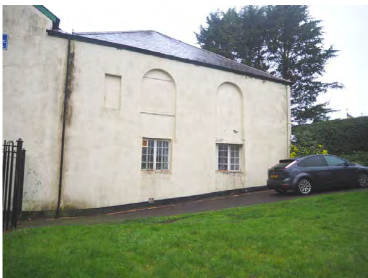
Fig 15: East elevation incorporates concealed windows openings at first floor level (also visible internally) and metal windows at ground floor level. Metal windows incorporate vent to kitchen.
