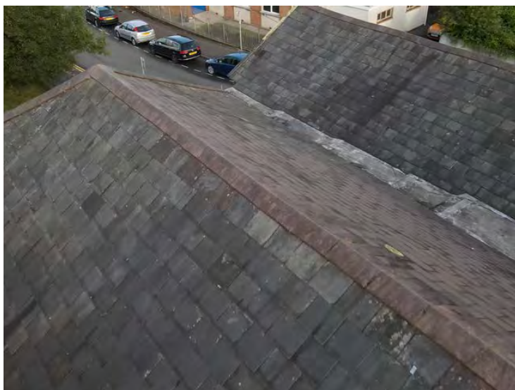
Fig 9: Staged lead valley connecting the hipped roof of the former Wesleyan Chapel (LHS of picture) and the gabled extension (top RHS of picture)
