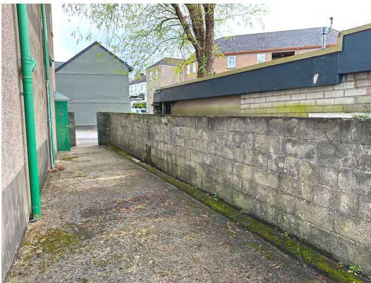
Fig 11: Access yard to west of building laid to concrete with drainage channel to perimeter.
