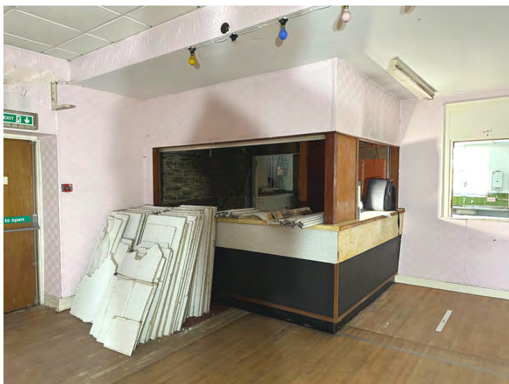
Fig 23: stained timber and melamine bar enclosure to north east corner of function room, leading to bar store and kitchen beyond.
