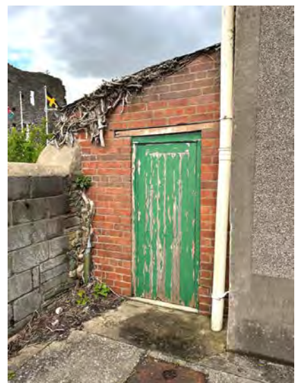
Fig 10: Lean to structure to north of former chapel with corrugated roof. Lean-to uses blockwork faced boundary wall within structure.
