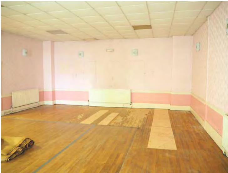
Fig 19: Former fire station entrance to east wall, Floor includes gentle slope towards former door. Modern panelled radiators fitted.
