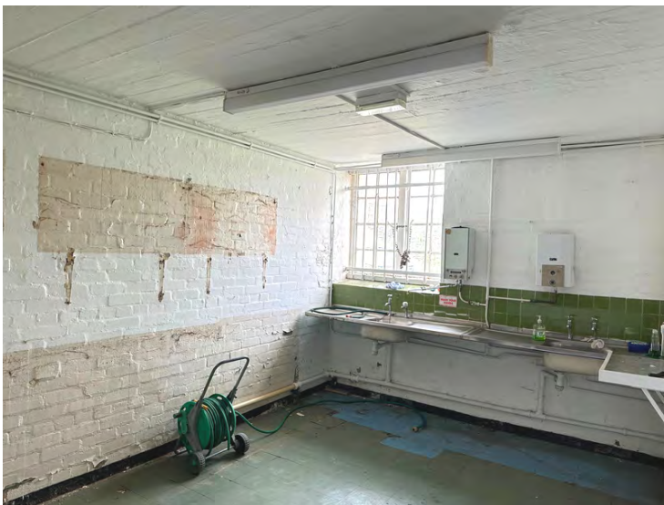
Fig 21: Kitchen adjacent to function space. Equipment removed with shuttered concrete ceiling, painted brick walls and vinyl tile floor evident. Metal windows to east elevation.
