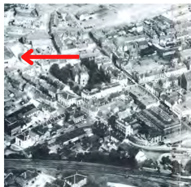
Fig 48: 1950's aerial image of Neath illustrating the building as a fire station (refer to large door opening in west elevation)
