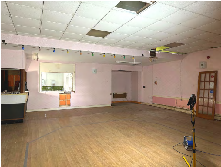
Fig 17: Main function space with access/view through serving hatch to kitchen. Surfaces include lay-in-grid ceiling, cementitious plaster walls/wallpaper finish and sprung timber floor.
