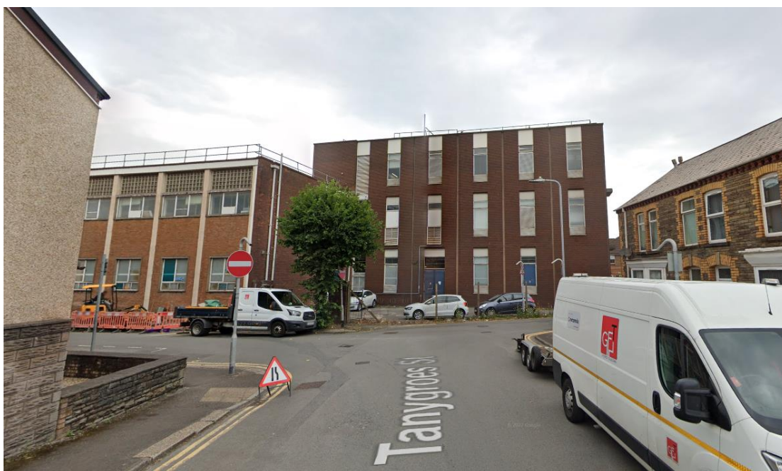
Short distance view of the site from Tan Y Groes Street
