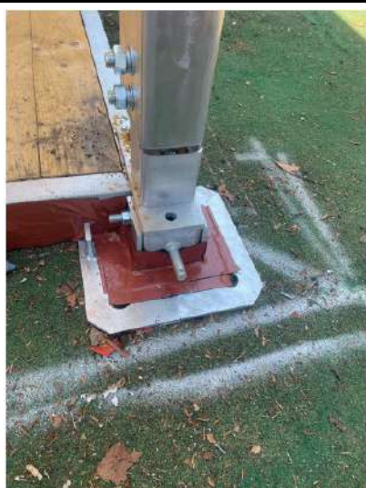
Photograph Three - View of continuous seal
