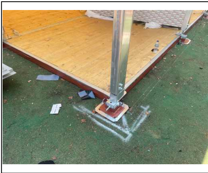
Additional sealed steel column.
