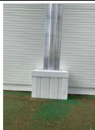
Photograph Six - Evidence that steel columns have now also been protected - with a PVC box.
