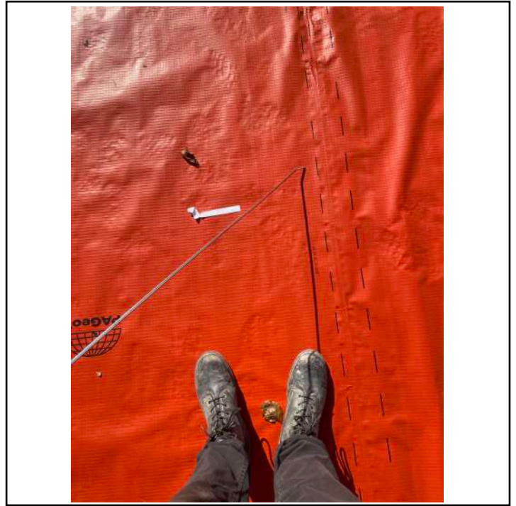
Air lance test to welded lap.
