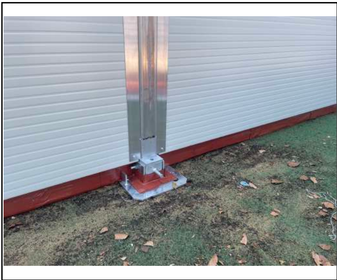
Additional sealed steel column.
