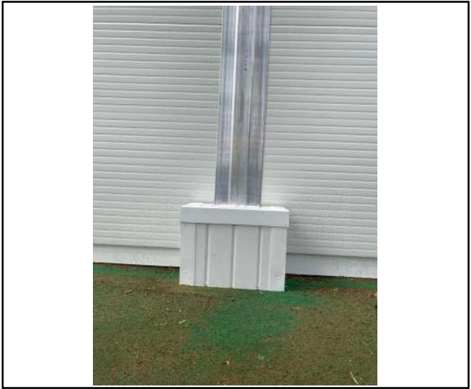
Steel column protected.
