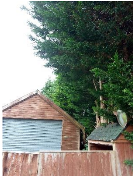
Trees overhanging existing garage
