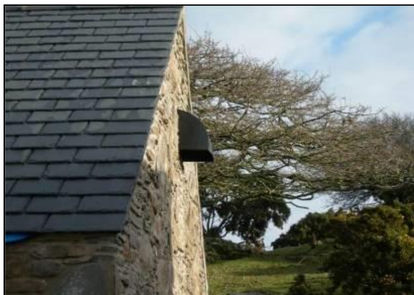
Example of a cowled hood for horseshoe bat access
