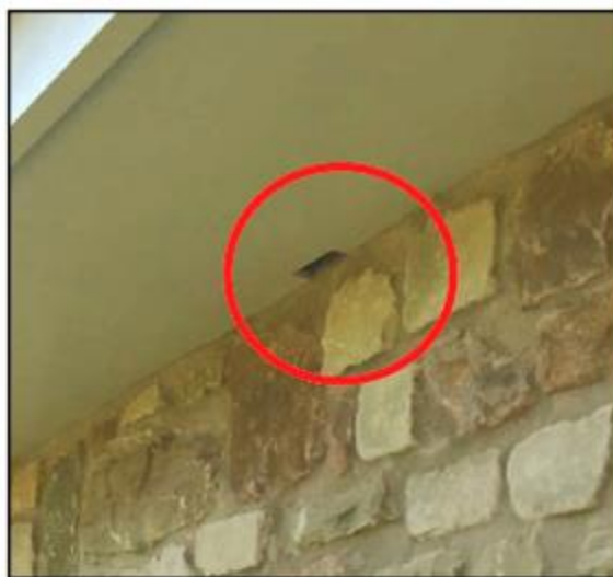
Below: Examples of soffit gaps.
