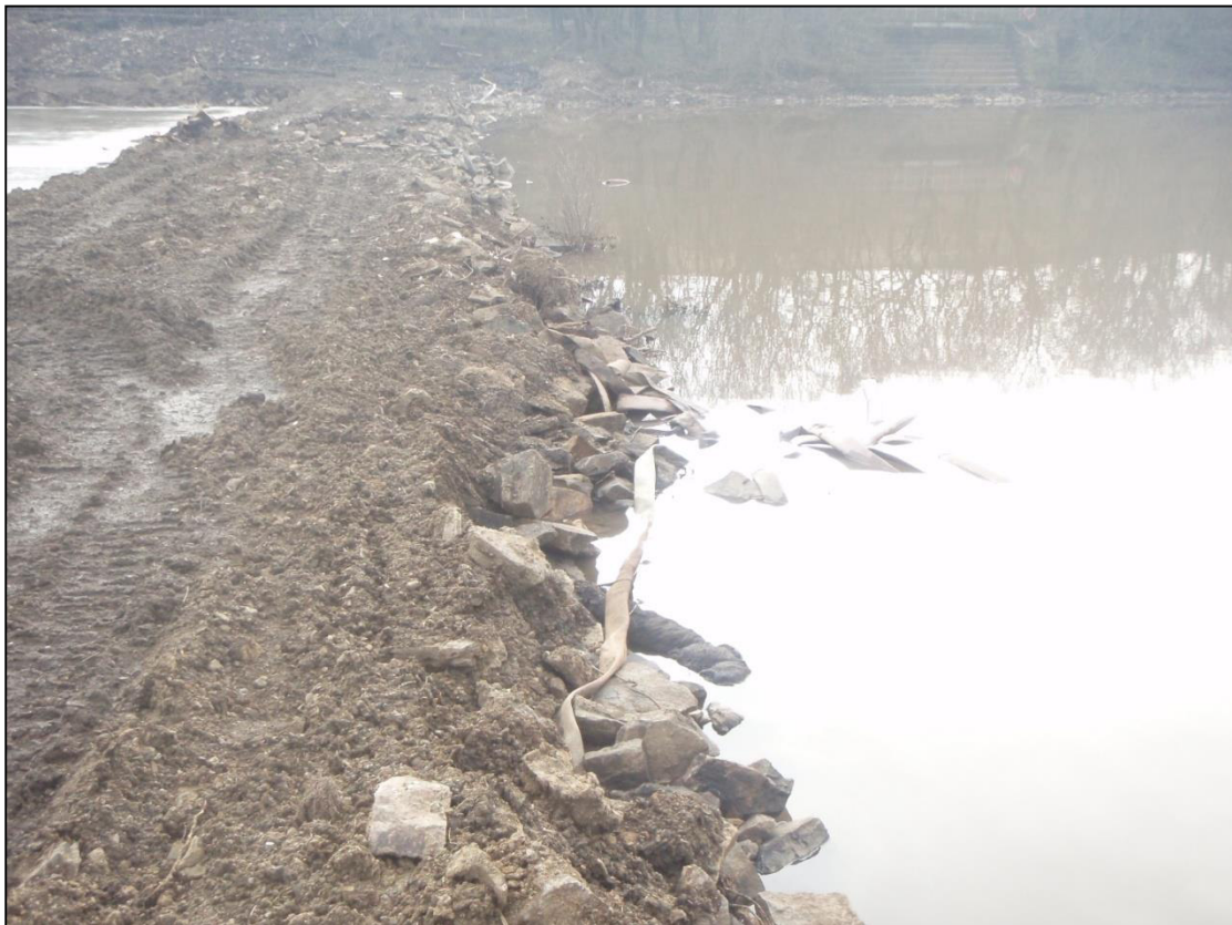
Photograph 4: North Site Reservoir Land Bridge remnant infrastructure clearance
