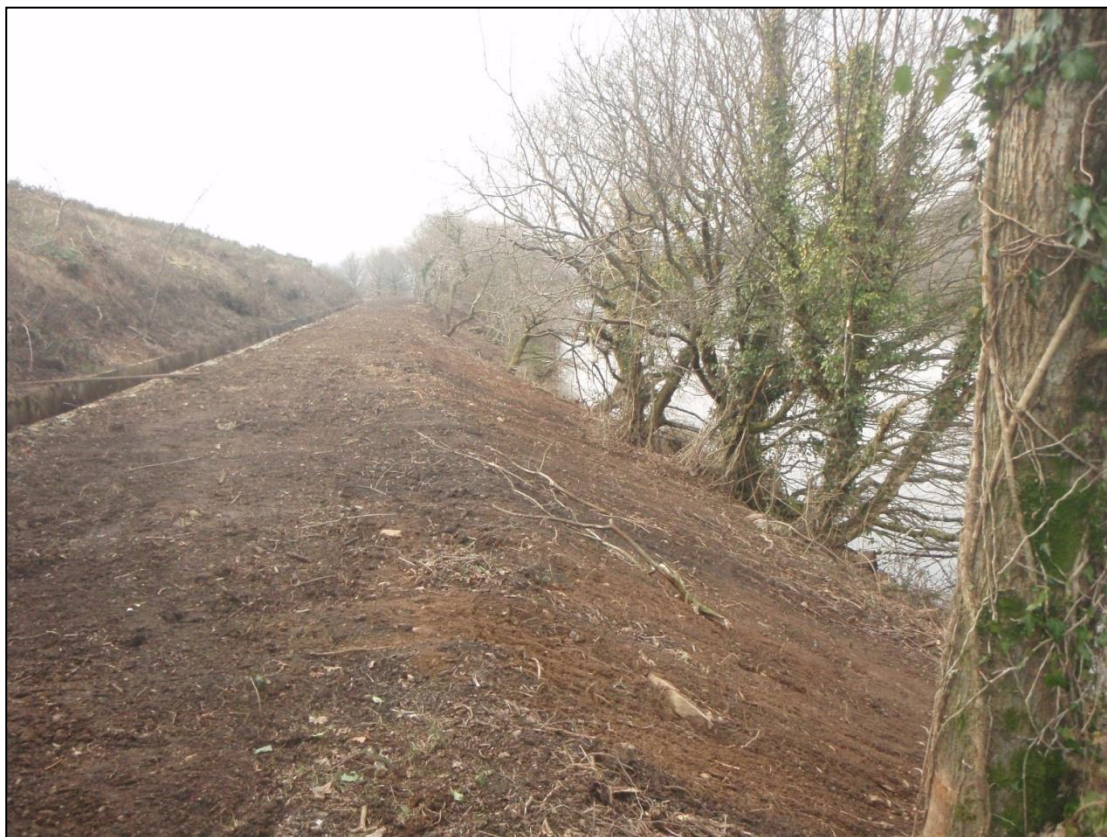
Photograph 5: North Site Reservoir remnant infrastructure clearance (Southern Bank looking west)
