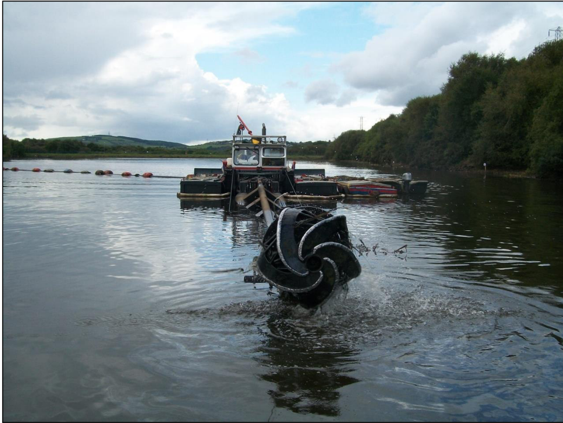
Photograph 1: Dredging Unit on Reservoir
