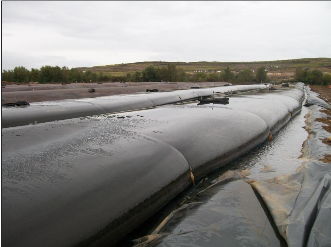
Photograph 3: Geotube dewatering sludge dredged from the reservoir
