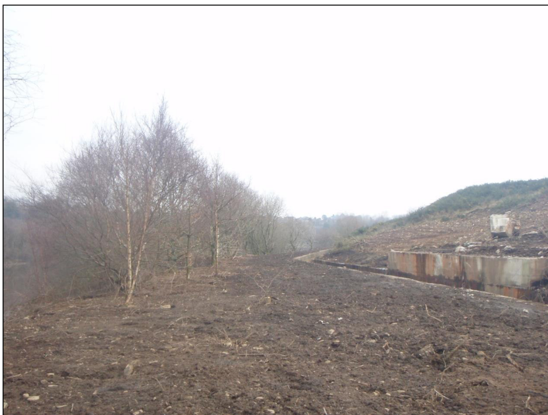
Photograph 6: North Site Reservoir remnant infrastructure clearance (Southern Bank looking east)
