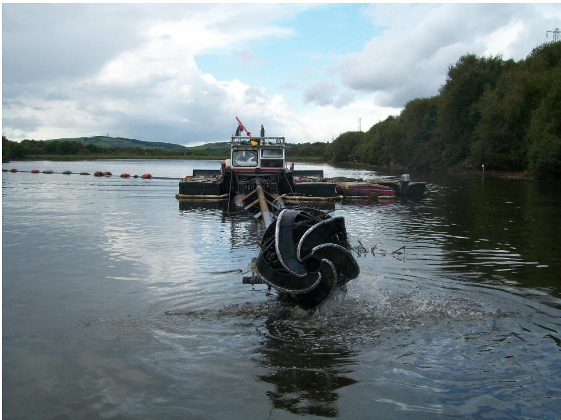
Photograph 8: Dredging Unit on Reservoir
