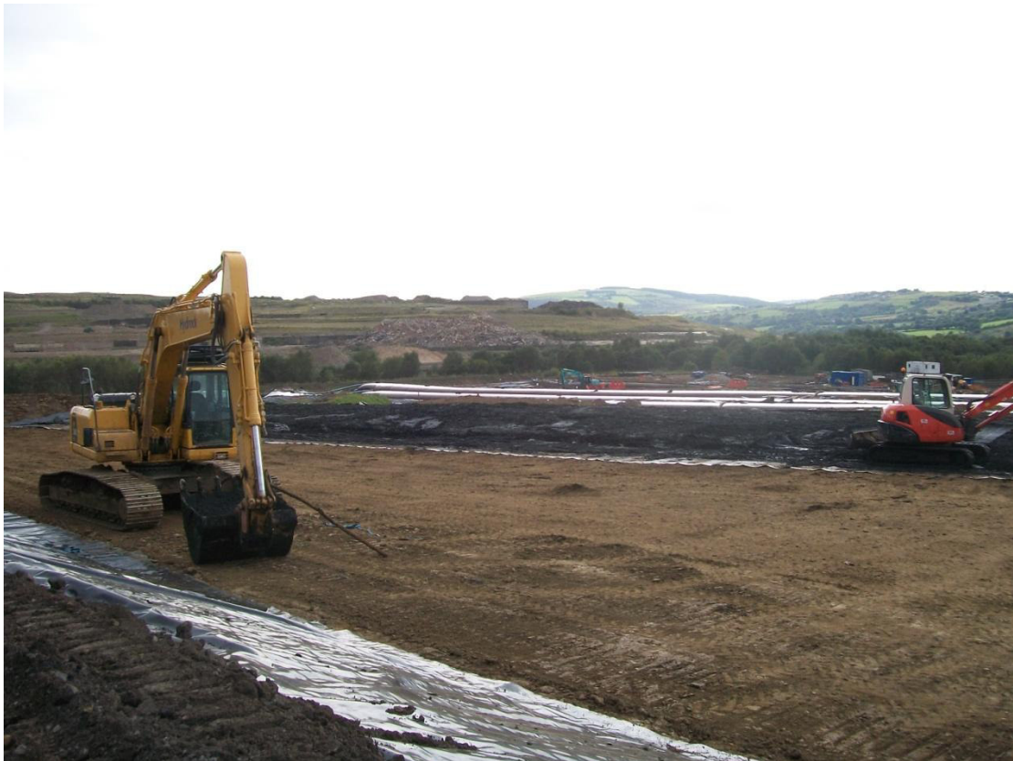
Photographs 7: Creation of a lined treatment area
