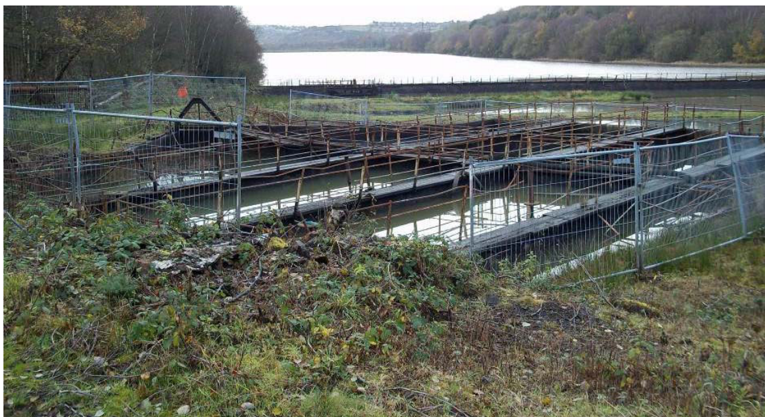
Photograph 6 – Separators prior to Demolition
