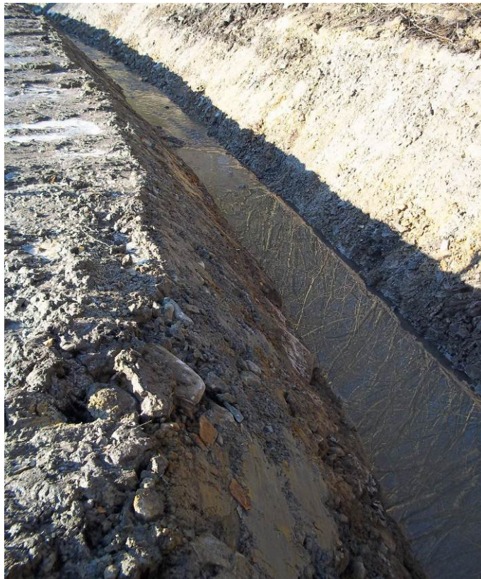
Photograph 2 – Motorway Drainage Diversion
