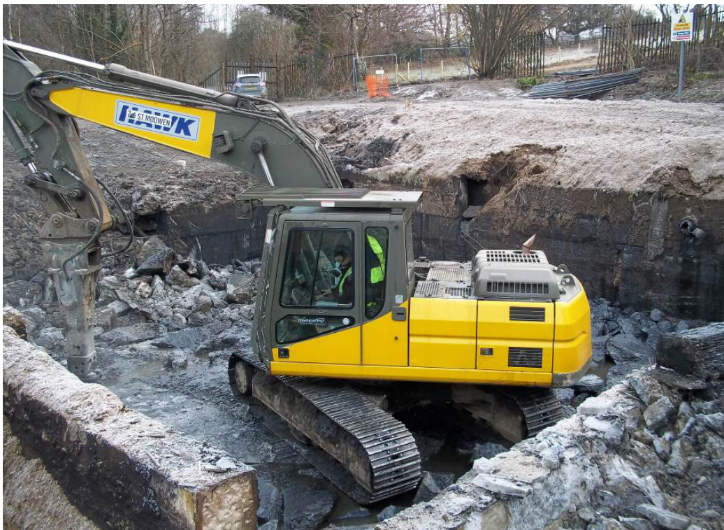
Photograph 9 – Demolition of the base following sludge removal
