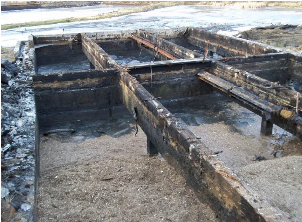
Photograph 7 – Mixing and removal of material within the separators
