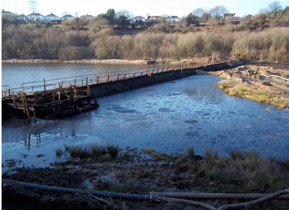
Photograph 5 – Low permeability bund, in the top right, created within East Bay
