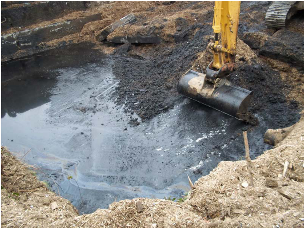
Photograph 8 – Scraping of concrete base of separators
