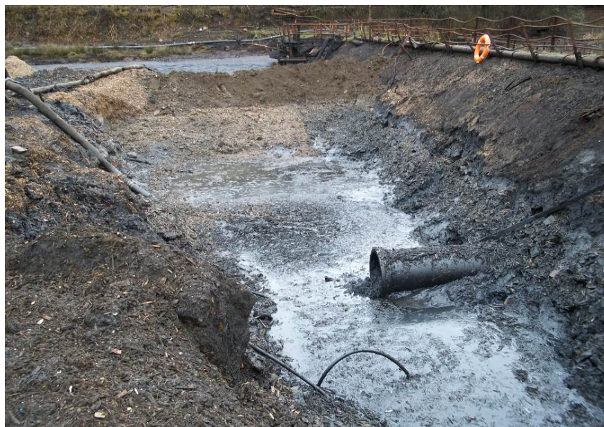
Photograph 4 – Low level pipe linking East Bay to NSR
