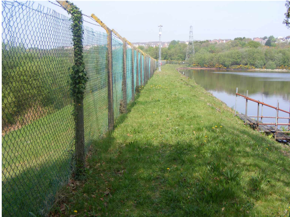
View looking north west along the crest of the dam
