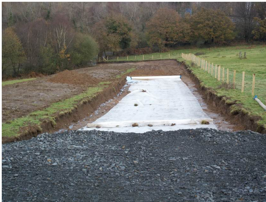
Photograph 1 – East Bay Access Road
