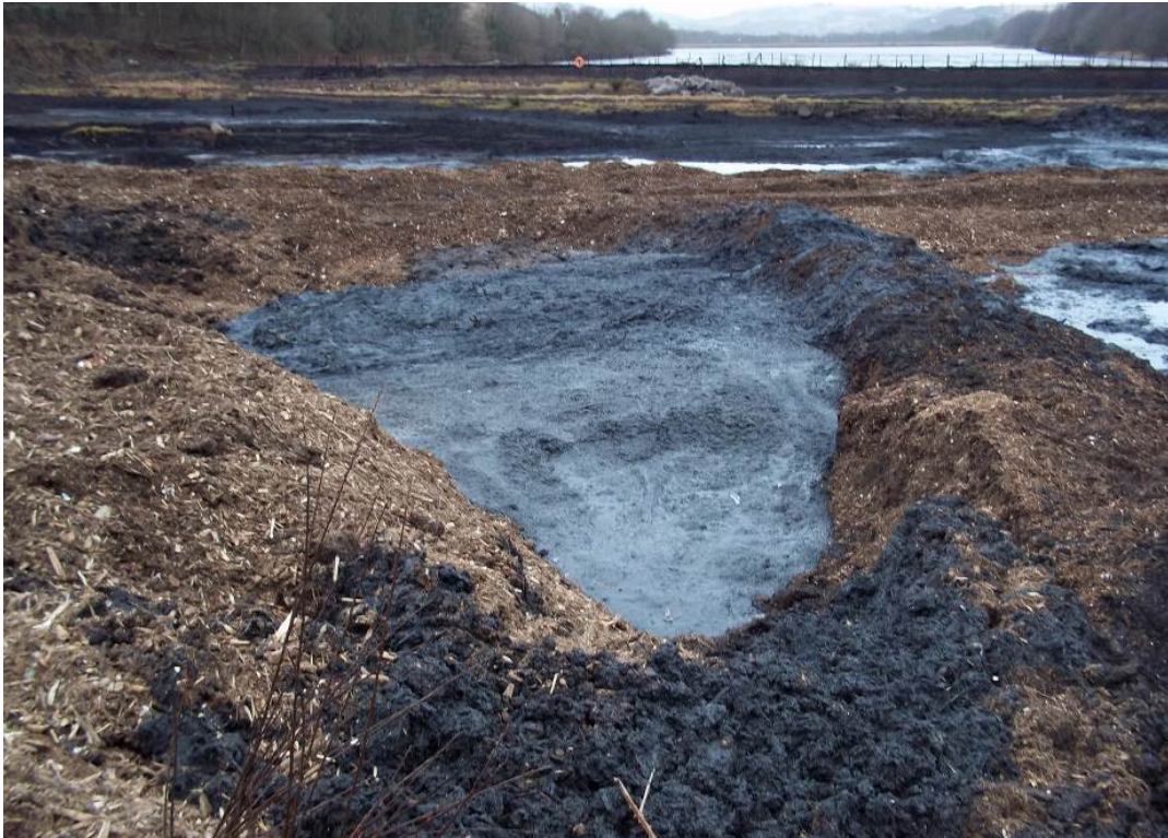
Photograph 11 – Hydrocarbon Impacted material within mixing bund at eastern section of East Bay
