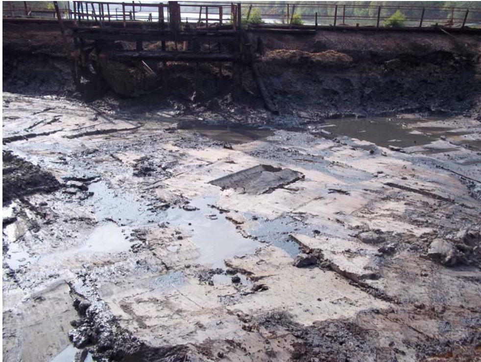
Photograph 22 – Southern section of Section 3 after the removal of hydrocarbon impacted material
