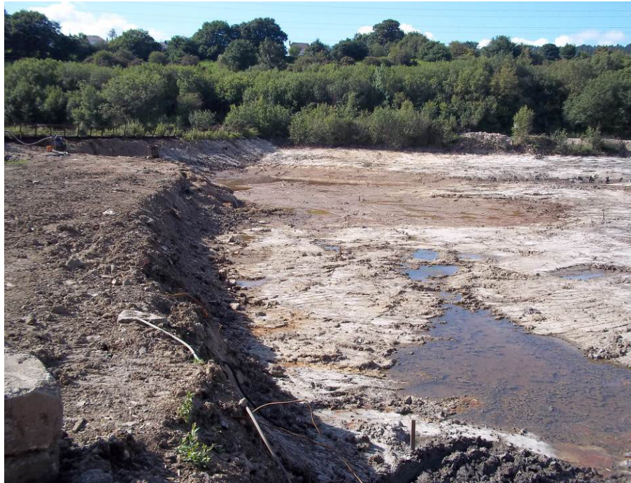
Photograph 18 – Section 2 following completion of the removal of hydrocarbon impacted material
