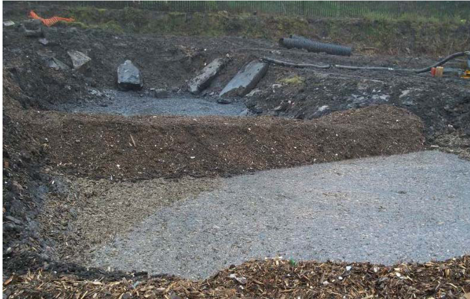
Photograph 20 – Settlement lagoon created at southern edge of Section 2
