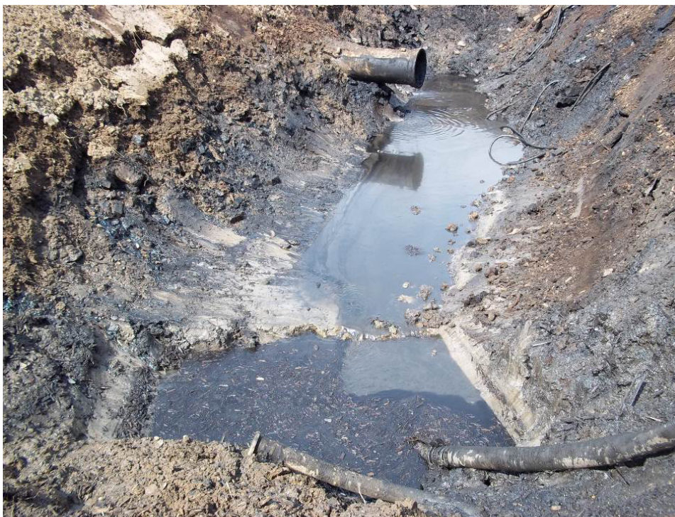
Photograph 24 – Northern area of Section 3 the removal of hydrocarbon impacted material
