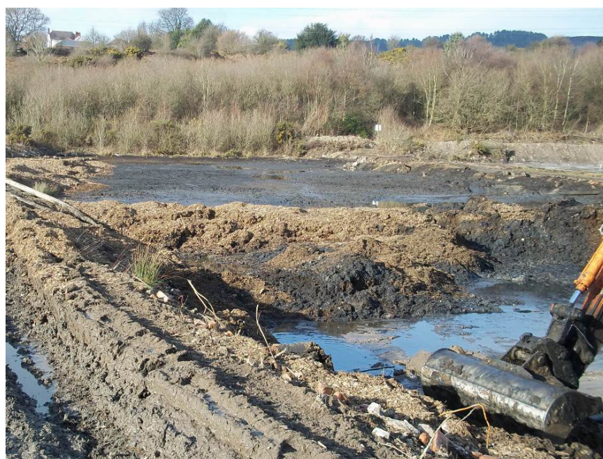
Photograph 16 – Section 2 of East Bay at start of removal process of hydrocarbon impacted material
