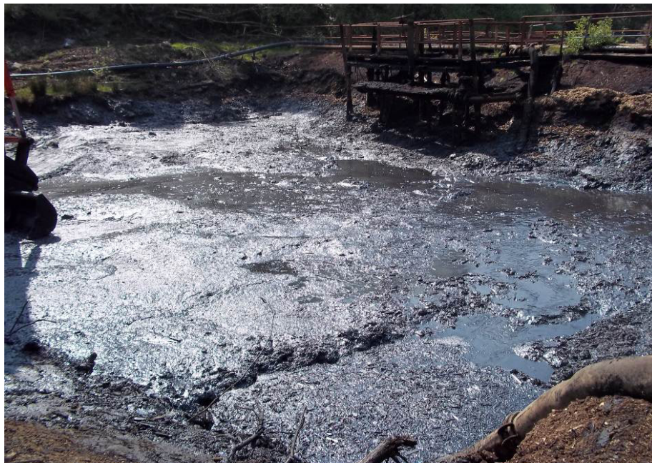
Photograph 21 – Southern area of Section 3 following de-watering but prior to the removal of hydrocarbon impacted material
