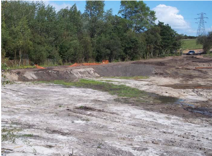
Photograph 14 – Band of organic material encountered at the base of East Bay (highlighted by vegetation growth)
