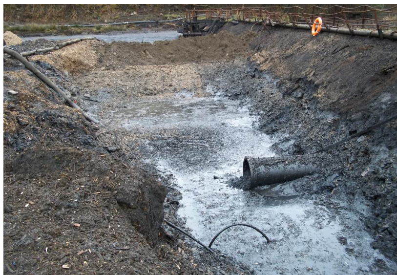
Photograph 19 – Section 3 divided into two work areas, note connecting pipework protruding from the NSR dam
