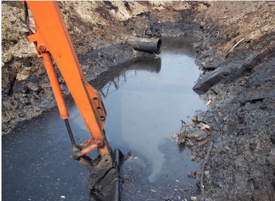
Photograph 24 – Northern area of Section 3 the removal of hydrocarbon impacted material
