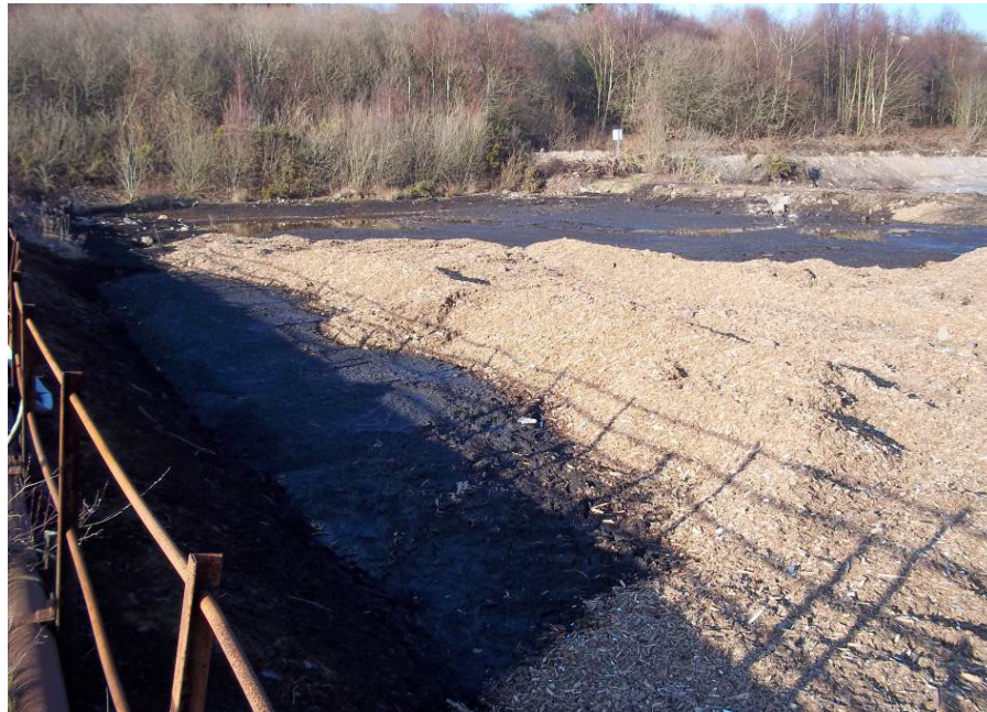
Photograph 15 – Wood fines bund created along dam between NSR and East Bay
