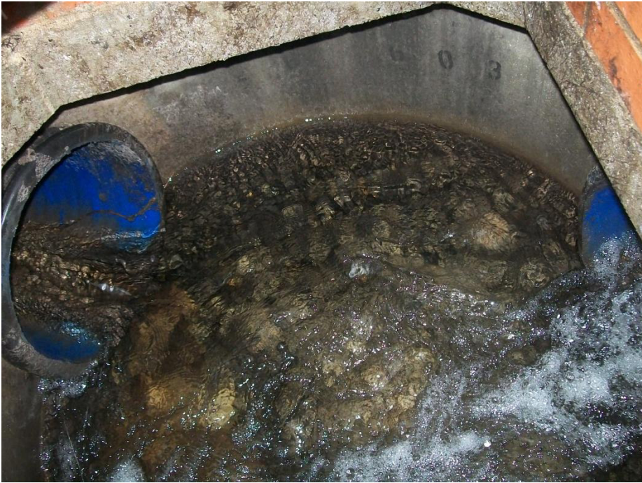
Plate 1. Manhole 016. M4 drainage manhole flow right to left.
