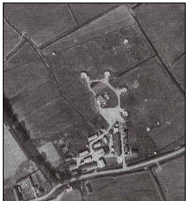
Above: Slade Green's HAA battery, Dartford showing typical size and layout of the installation.
