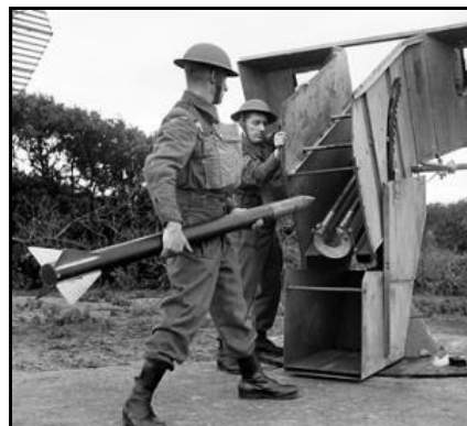
Home Guard soldiers load an anti-aircraft rocket at a 'Z' Battery
