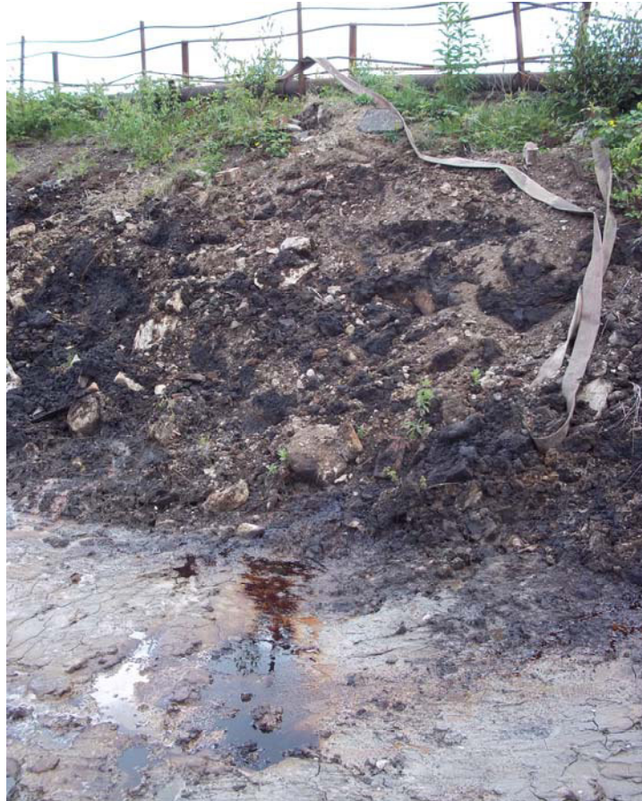
Photograph 28 – Hydrocarbon seepage noted from dam between East Bay and NSR
