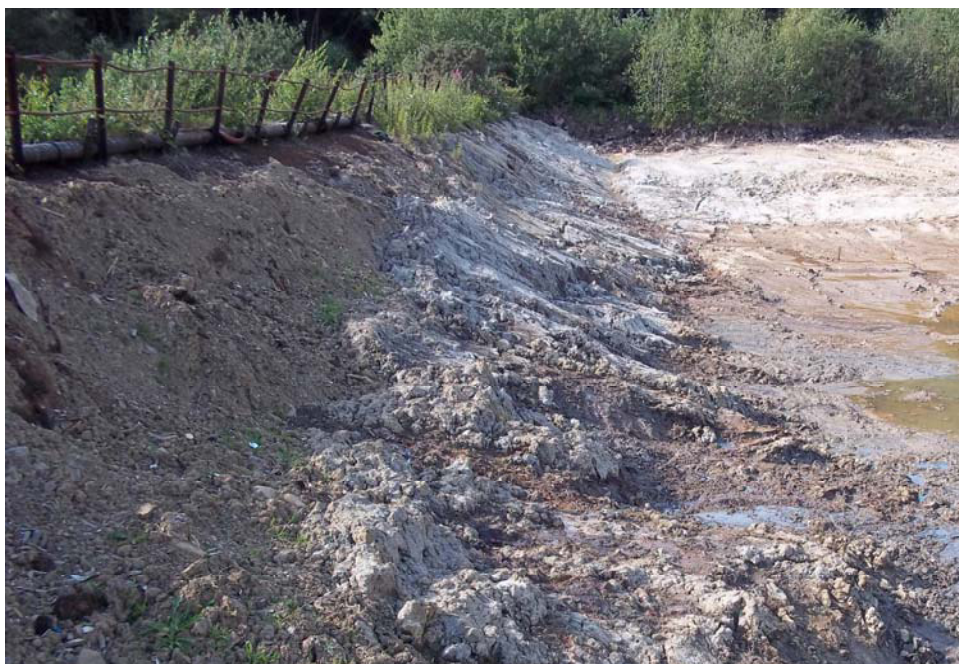
Photograph 29 – Clay material placed against NSR Dam prior to inundation
