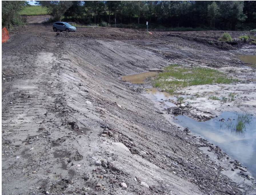
Photograph 31 – Eastern embankment following removal of potentially hydrocarbon impacted material and re-profiling
