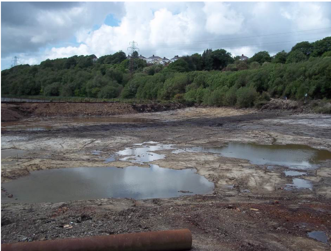
Photograph 27 – Central pier completely removed
