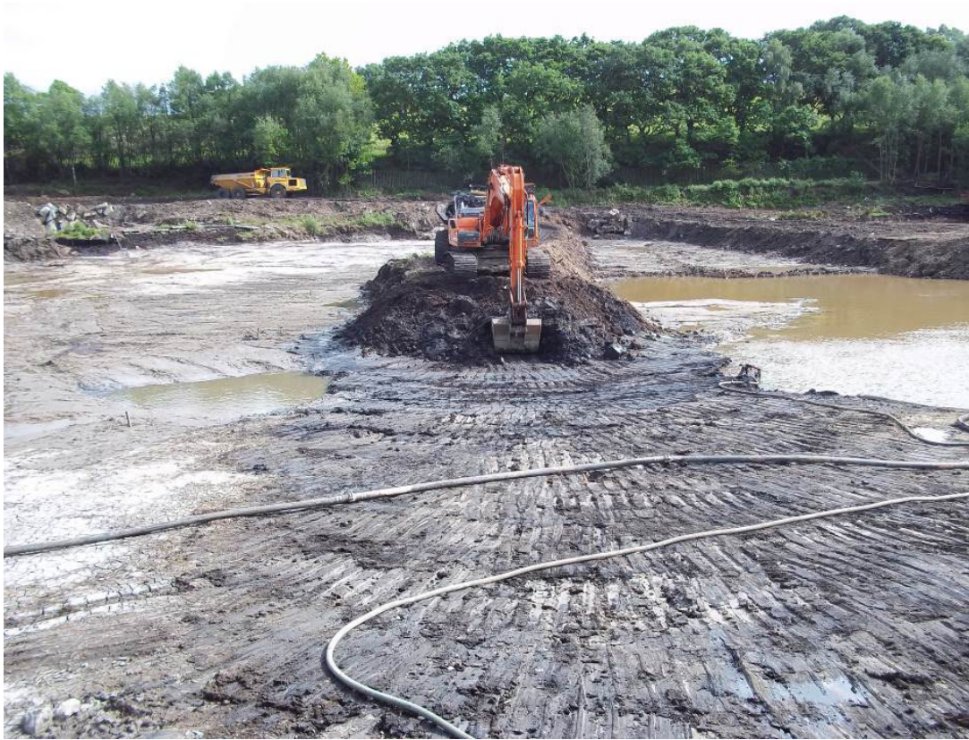
Photograph 26 – Central pier partially removed
