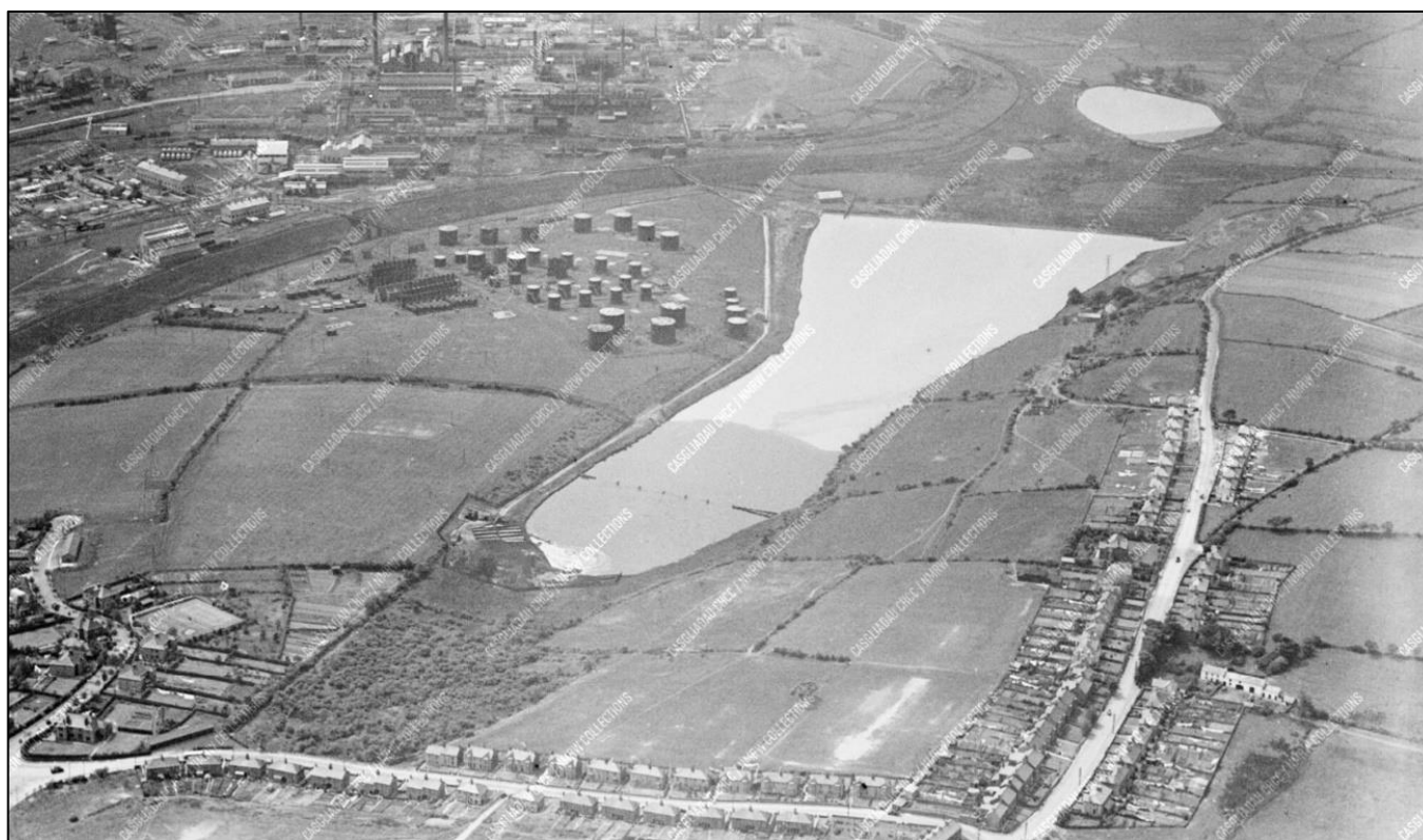
Image 3: NSR viewed from the north east
