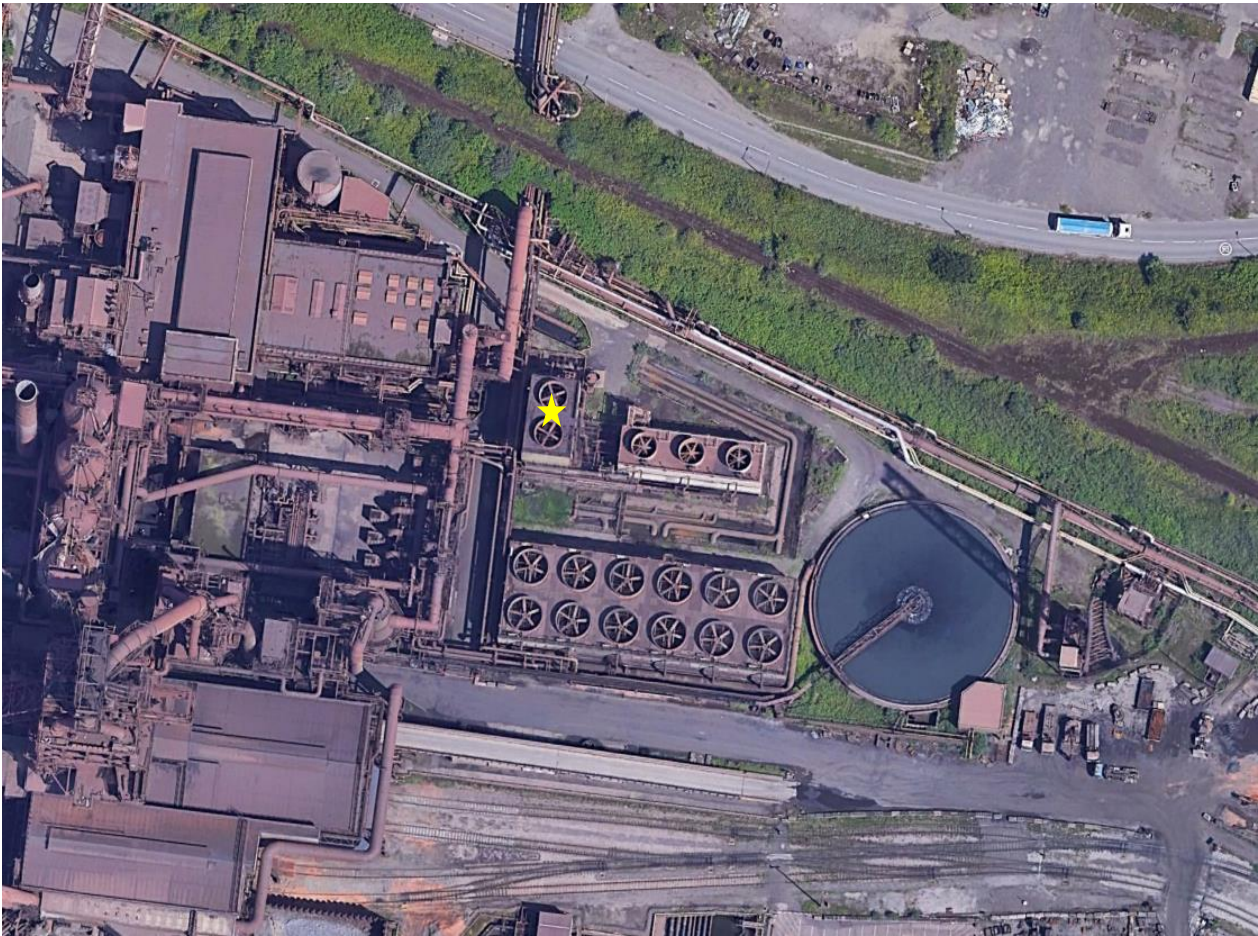
Figure 2: The Water Cooling Tower to be deconstructed (Google Earth).
