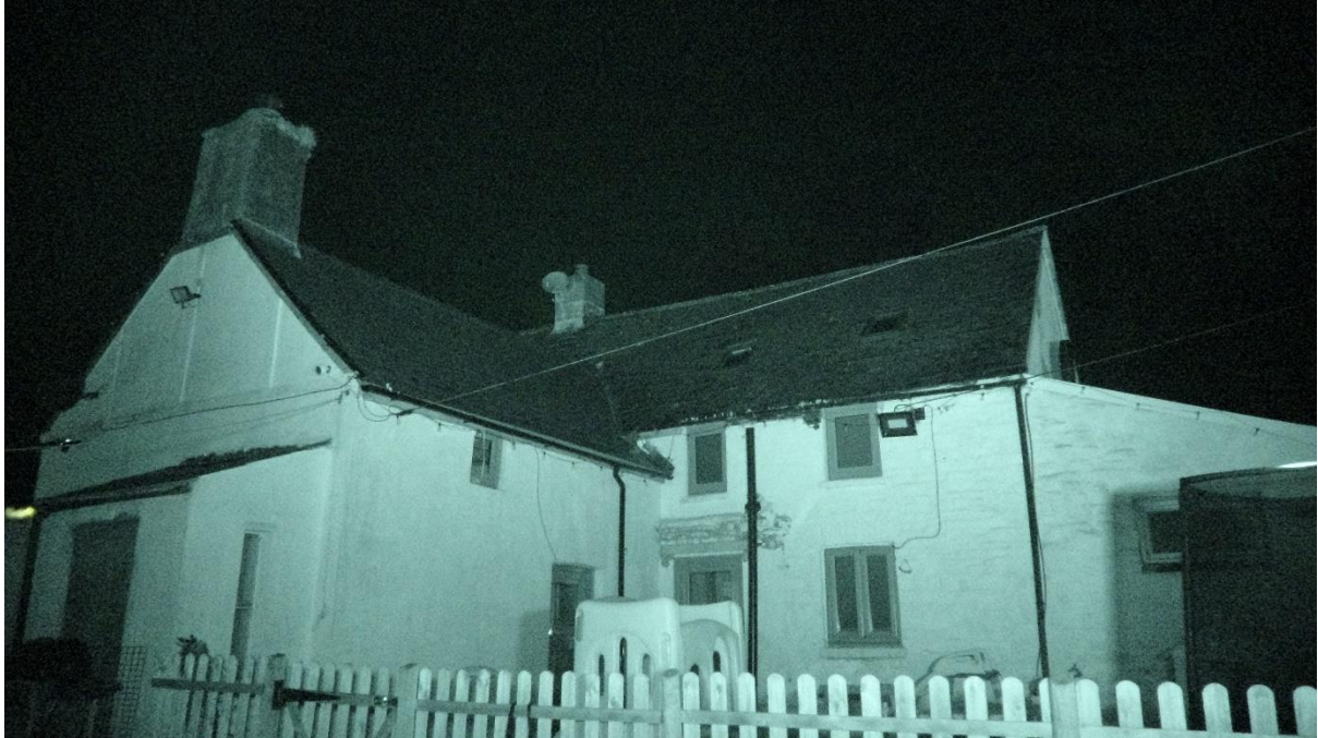
Photograph of the south east elevation at the darkest point of the surveys
