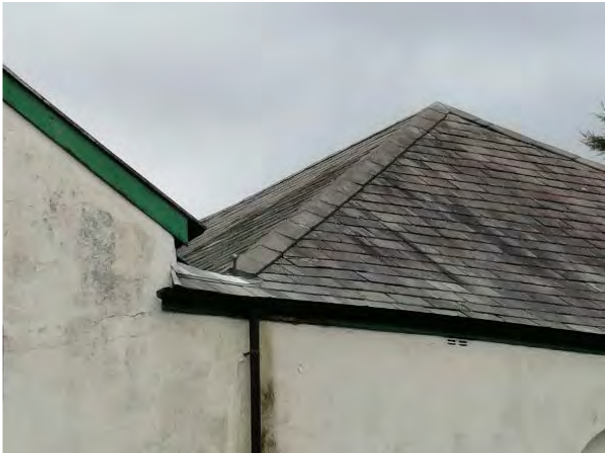
Photo 4 – Front Roof Profile
