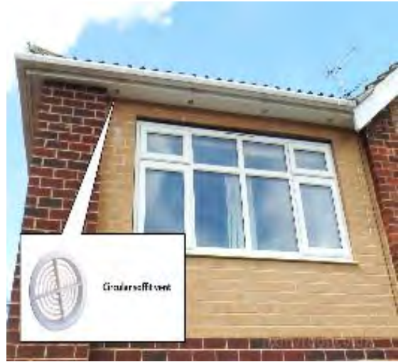
Figure 4 : Ventilation Soffit Boards
