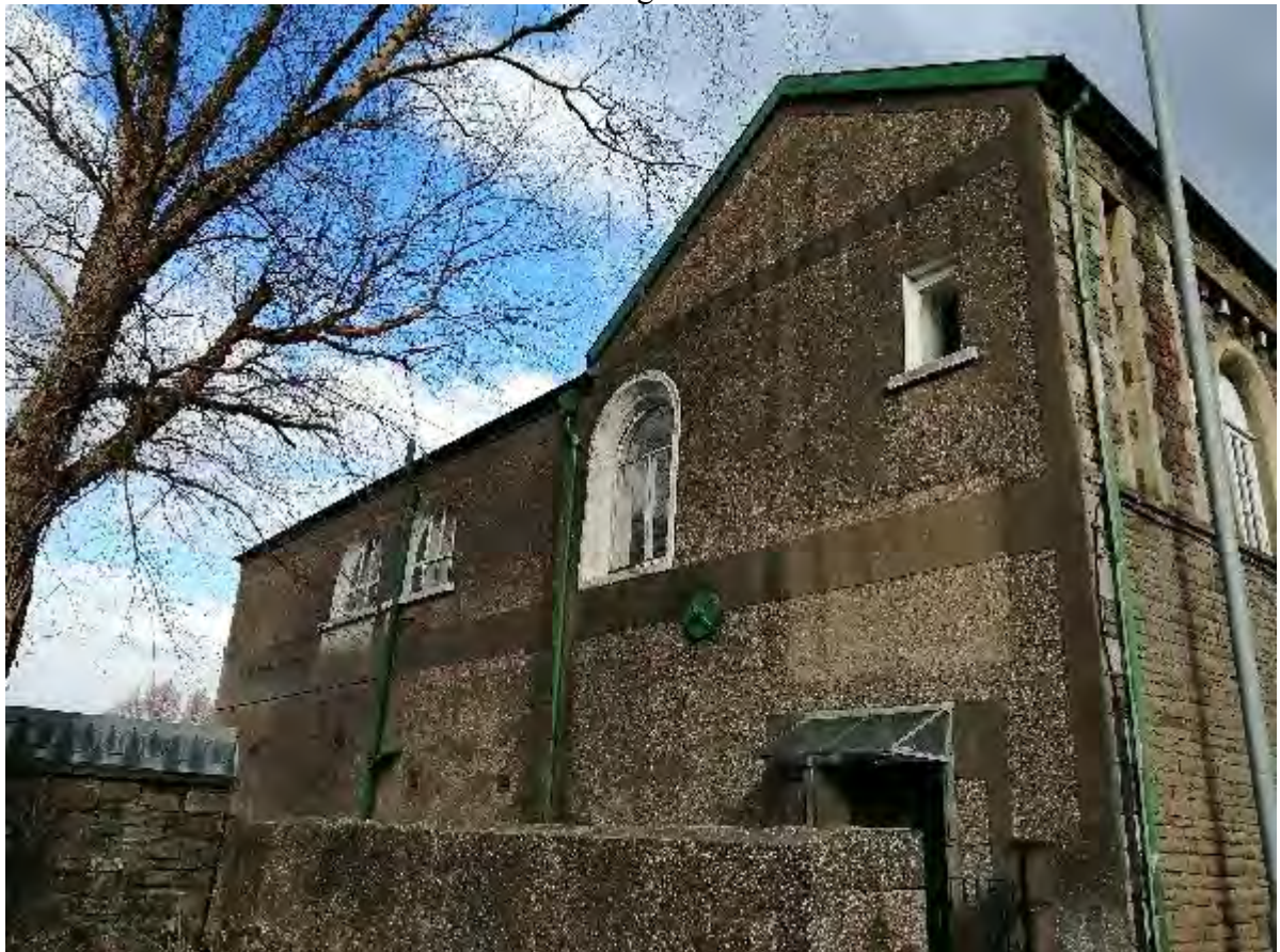
Photo 25 – Left Side Wall Elevation (Upper)
