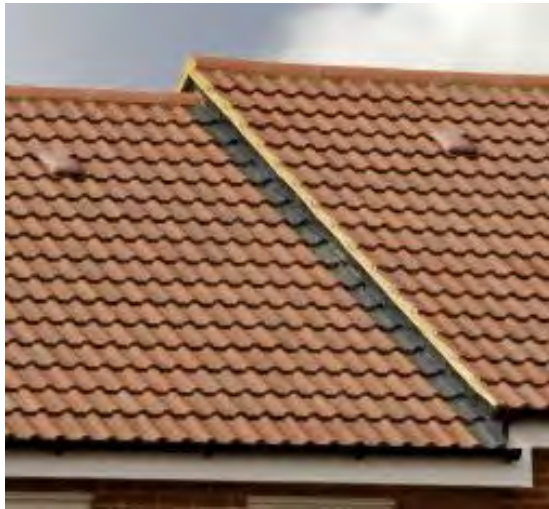
Figure 3 : Ventilation Roof Tiles
