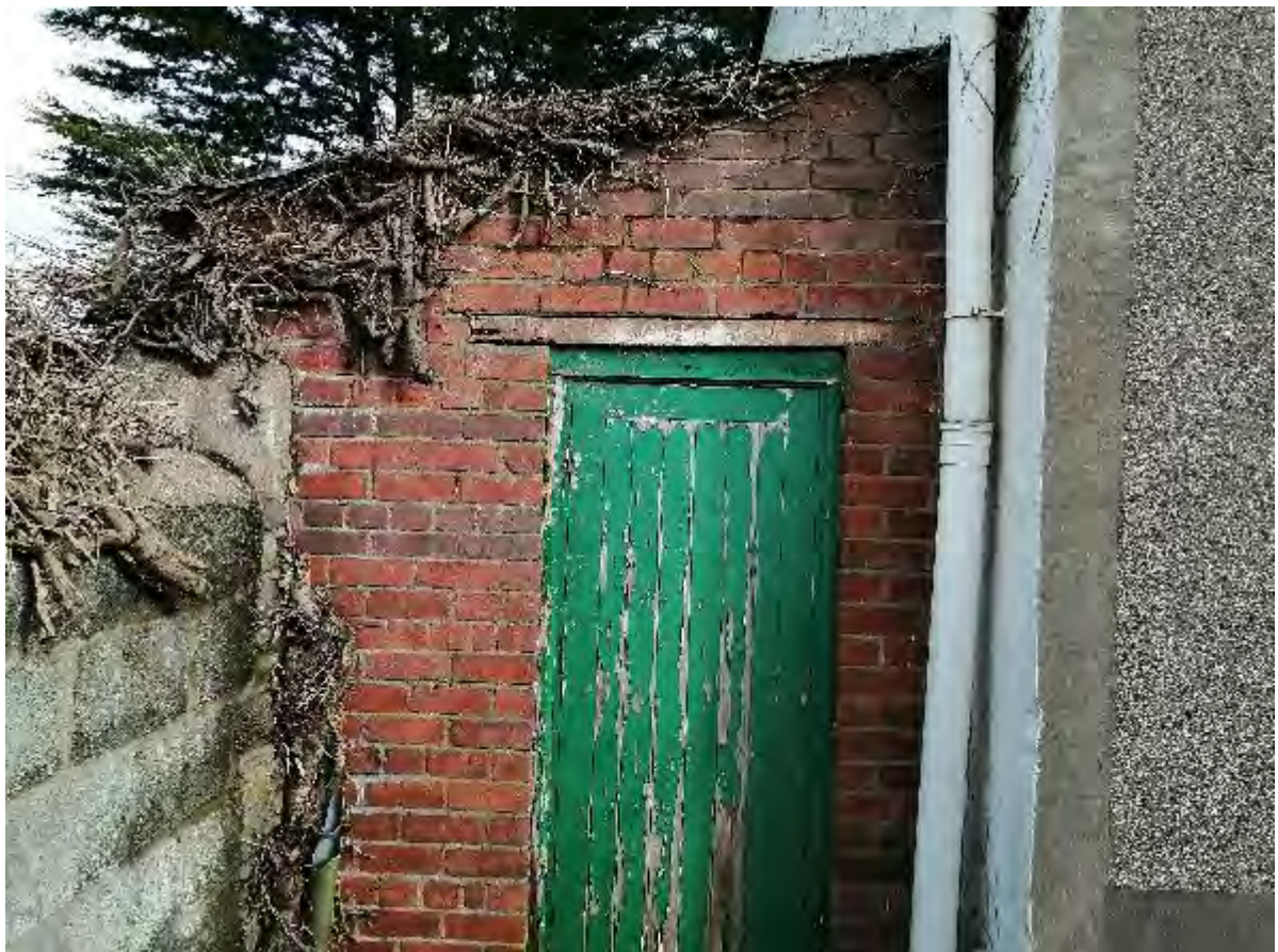
Photo 27 – Left Side Wall Elevation
