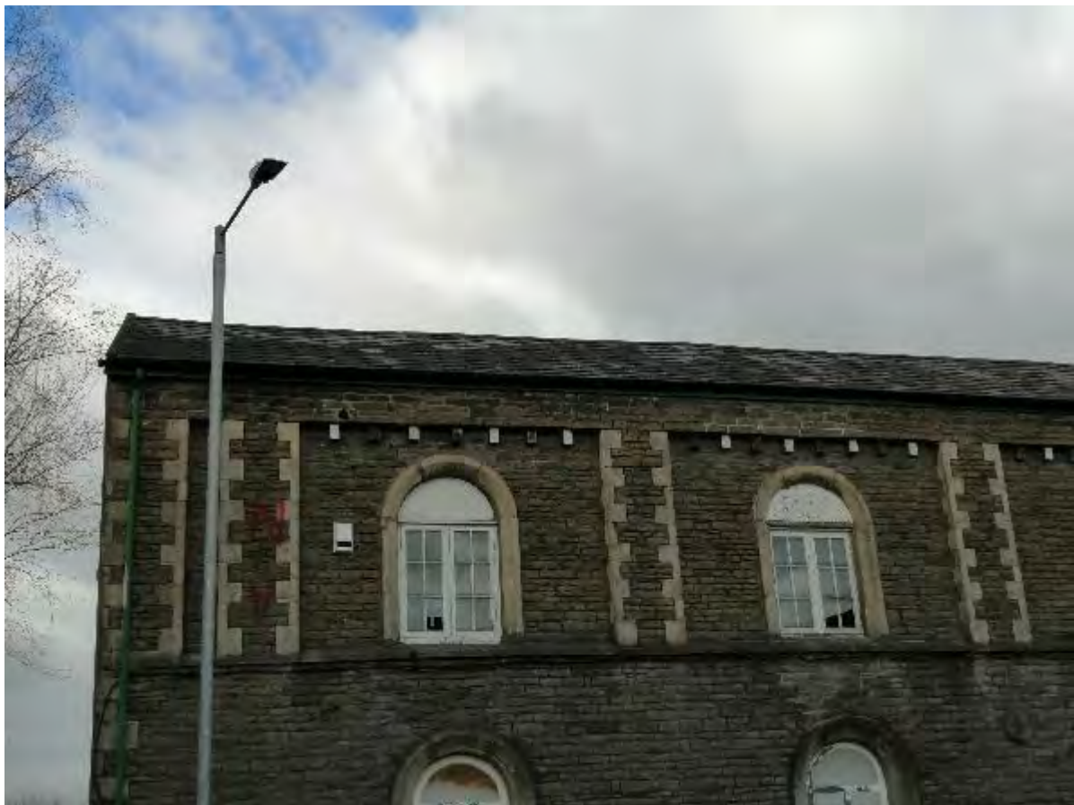
Photo 1 – Front Roof Profile (Left)
