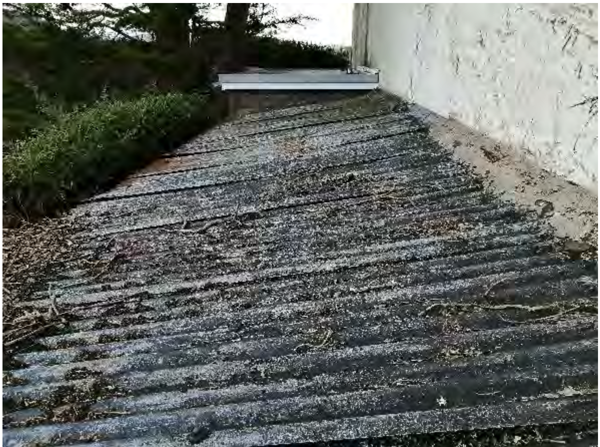
Photo 9 – Rear Roof Profile
