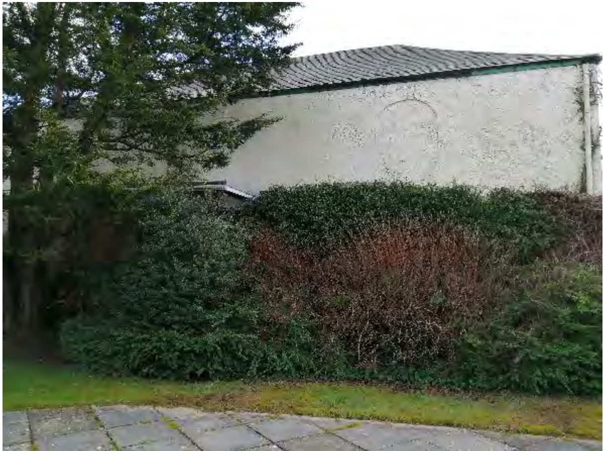
Photo 29 – Rear Wall Elevation (Upper)
