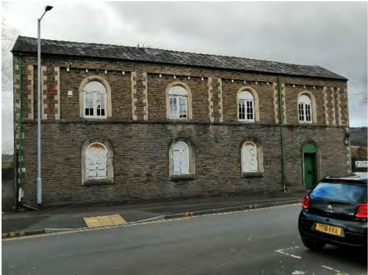
Photo 22 – Front Wall Elevation
