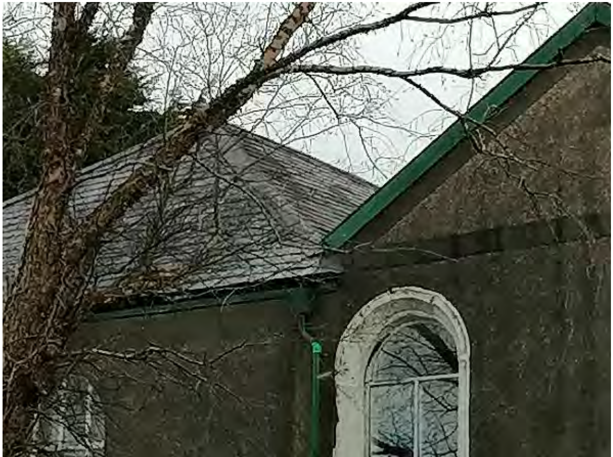
Photo 3 – Front Roof Profile
